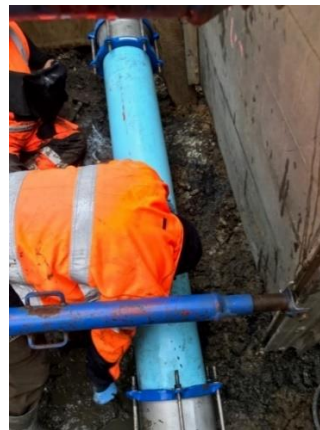
The repaired portion of the rising main
