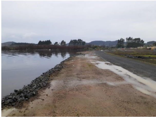
The dividing embankment between #1 Pond and the seepage pond
