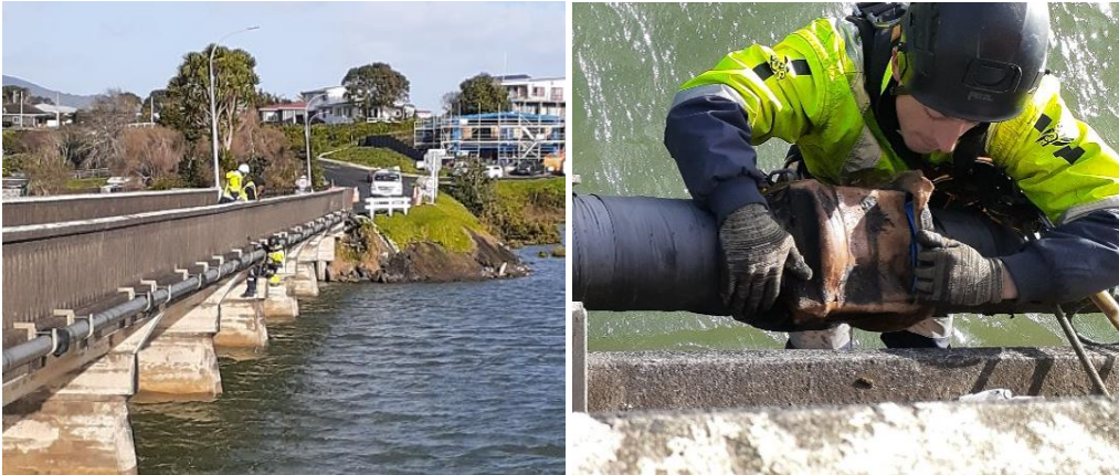
Abseilers carrying out gibault repair work
