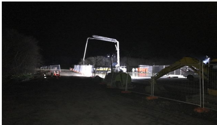
The second concrete pad pour for MABR tanks was completed at the end of July
