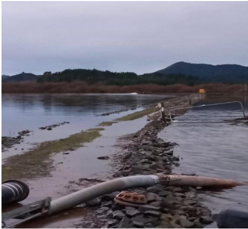
Dividing embankment between # 1 and # 2 ponds
