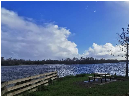
Picnic table installation, Ohinewai Boat Ramp
