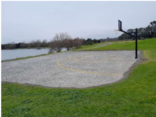
Basketball hoop installation, Lake Puketirini, Huntly
