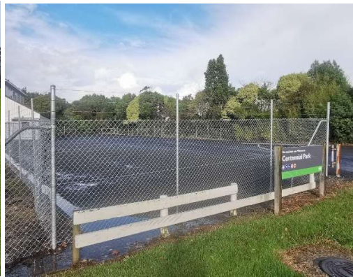
Fence installation, Centennial Park, Ngaruawahia
