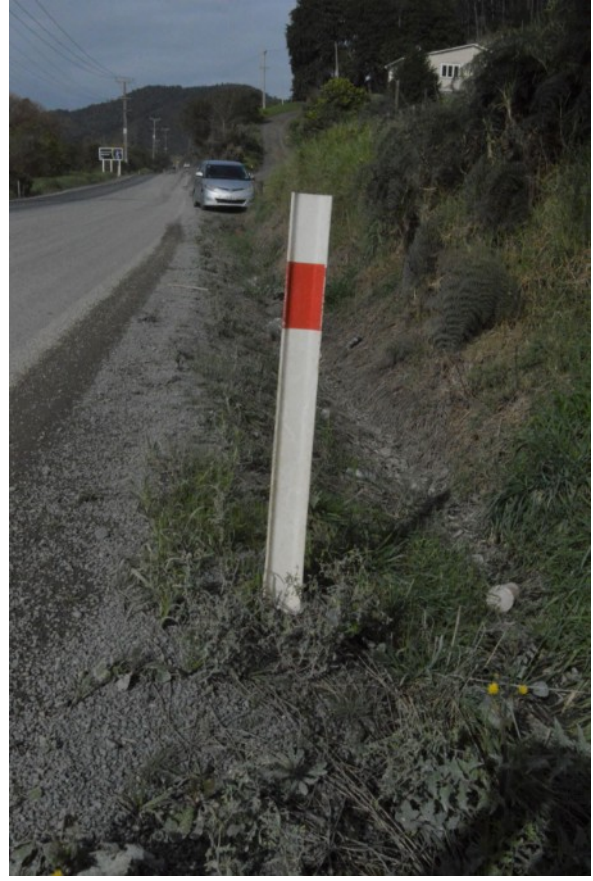
Example of dust and crud build up. This is either side of a road marker ~ 0.9km North of quarry One side completely non longer functioning as a marker!
