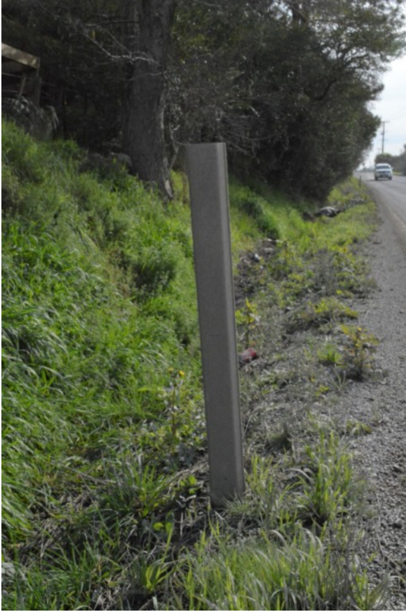
Example of dust and crud build up. This is either side of a road marker ~ 0.9km North of quarry One side completely non longer functioning as a marker!
