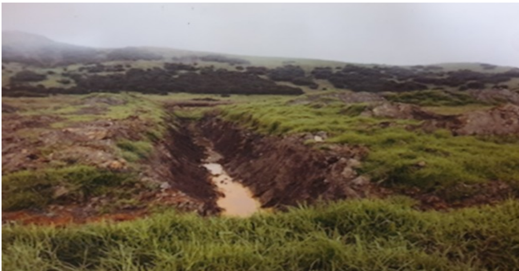
Illegal ditch created to drain a wetland
