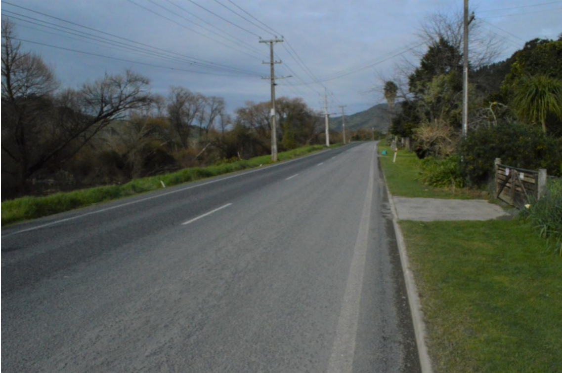
Example of dust and debris build up on Riverview ~1.5 km north of quarry. The dust trail was clearly visible until the roundabout 2.8?km away.
