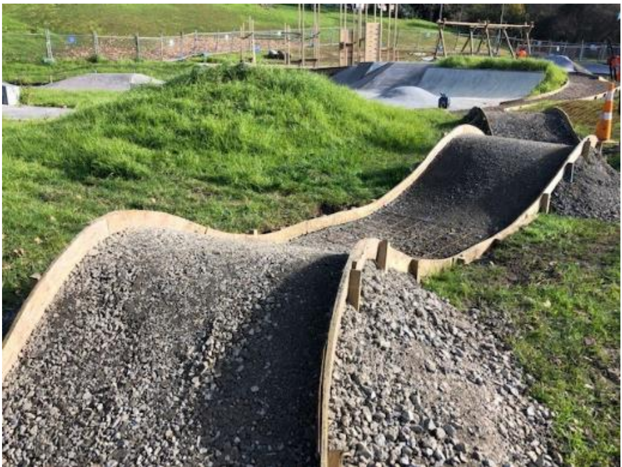
Pump track boxed ready for concreting
