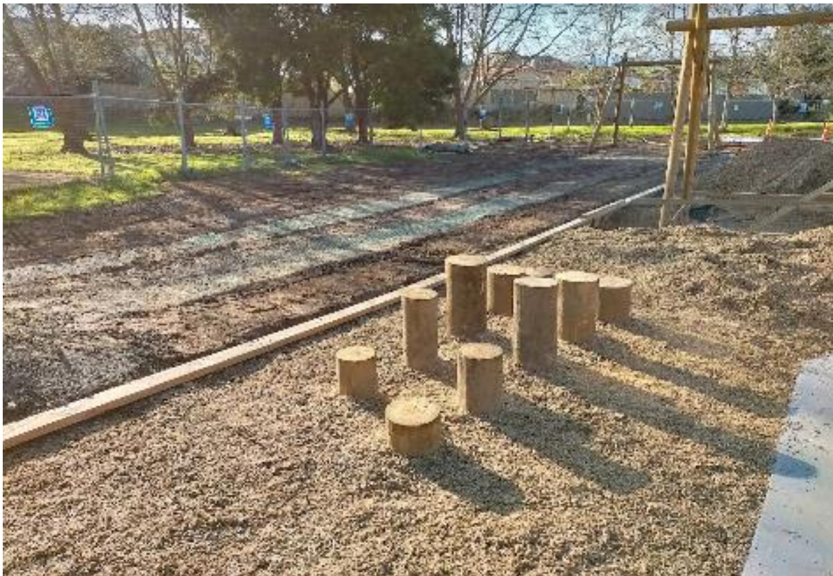
Stepping logs installed
