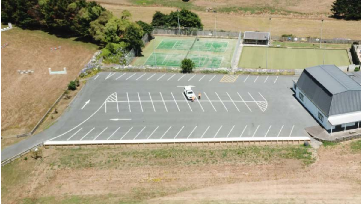
Te Akau Sports Complex Carpark Upgrade
