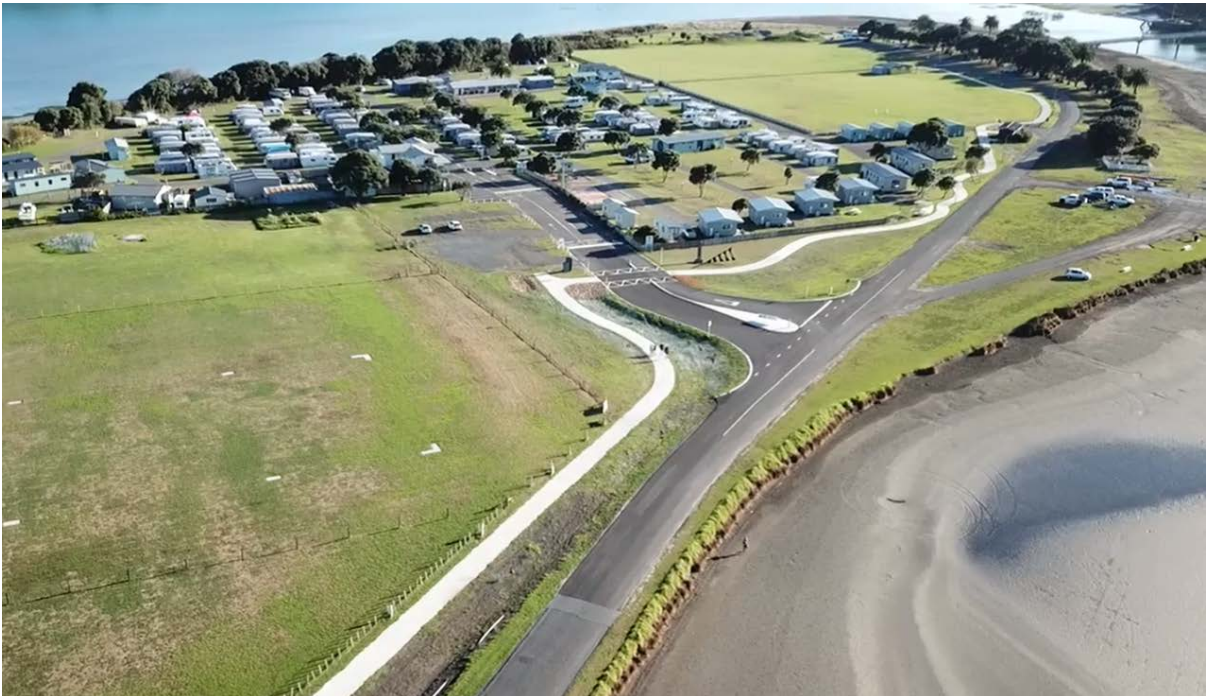
Papahua Walkway/Cycleway and Campground Entrance - Raglan
