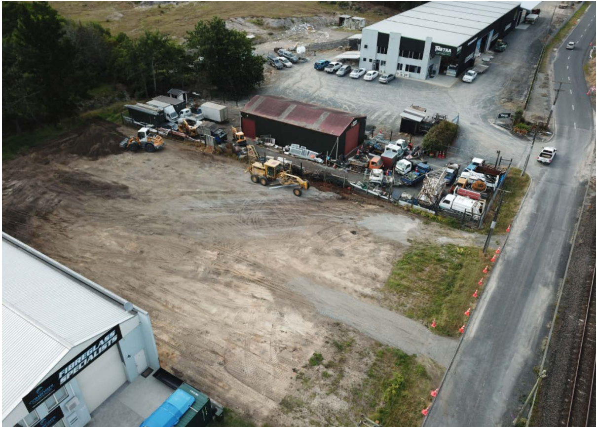
Tregoweth Lane Utilities Renewals and Relocation – Huntly
