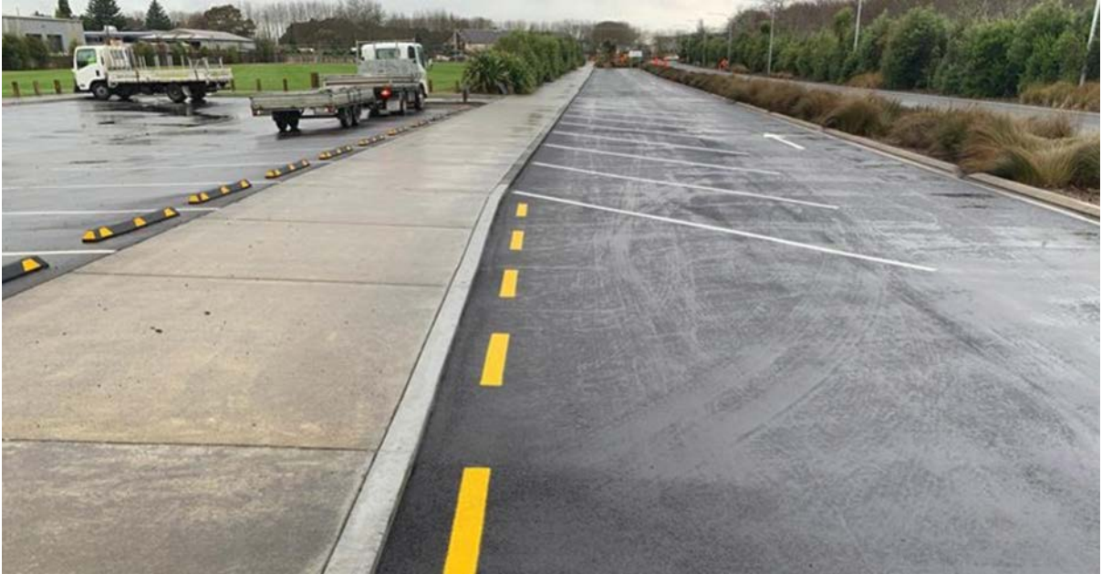
Wiremu Tamihana Drive Carpark Upgrade - Tamahere
