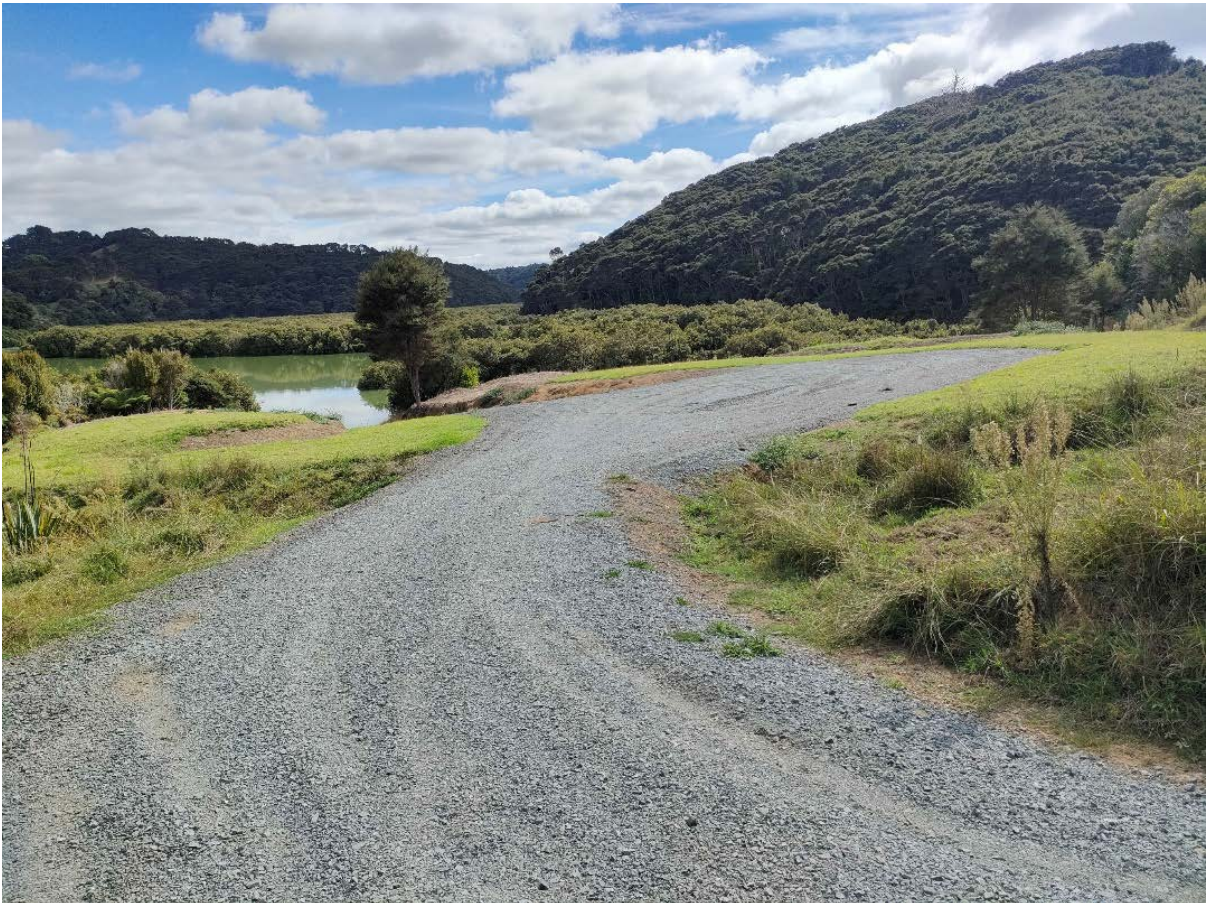
Waingaro Landing Carpark Upgrade
