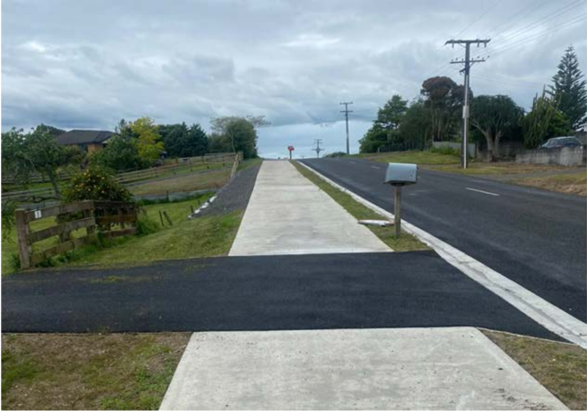
Travers Rd Walkway Extension, Te Kauwhata
