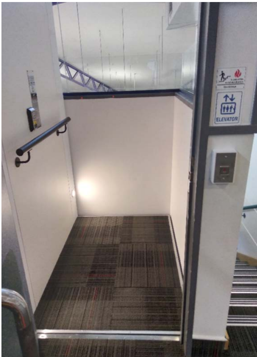
Huntly Library Lift Replacement
