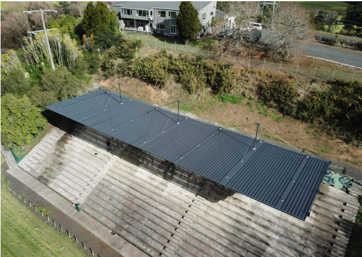
Huntly Grandstand Roof Replacement - Huntly
