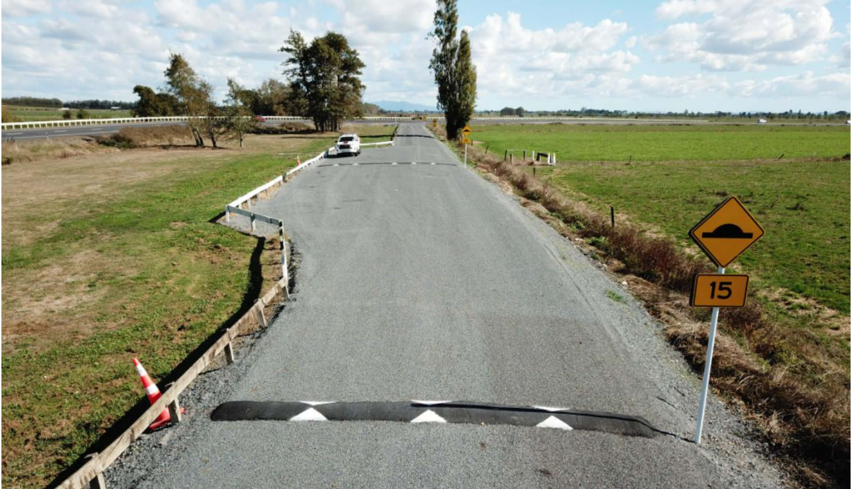
Piako Road Rest Area Carpark Upgrade
