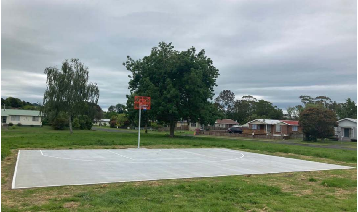
Brownlie Crescent Basketball Halfcourt – Huntly
