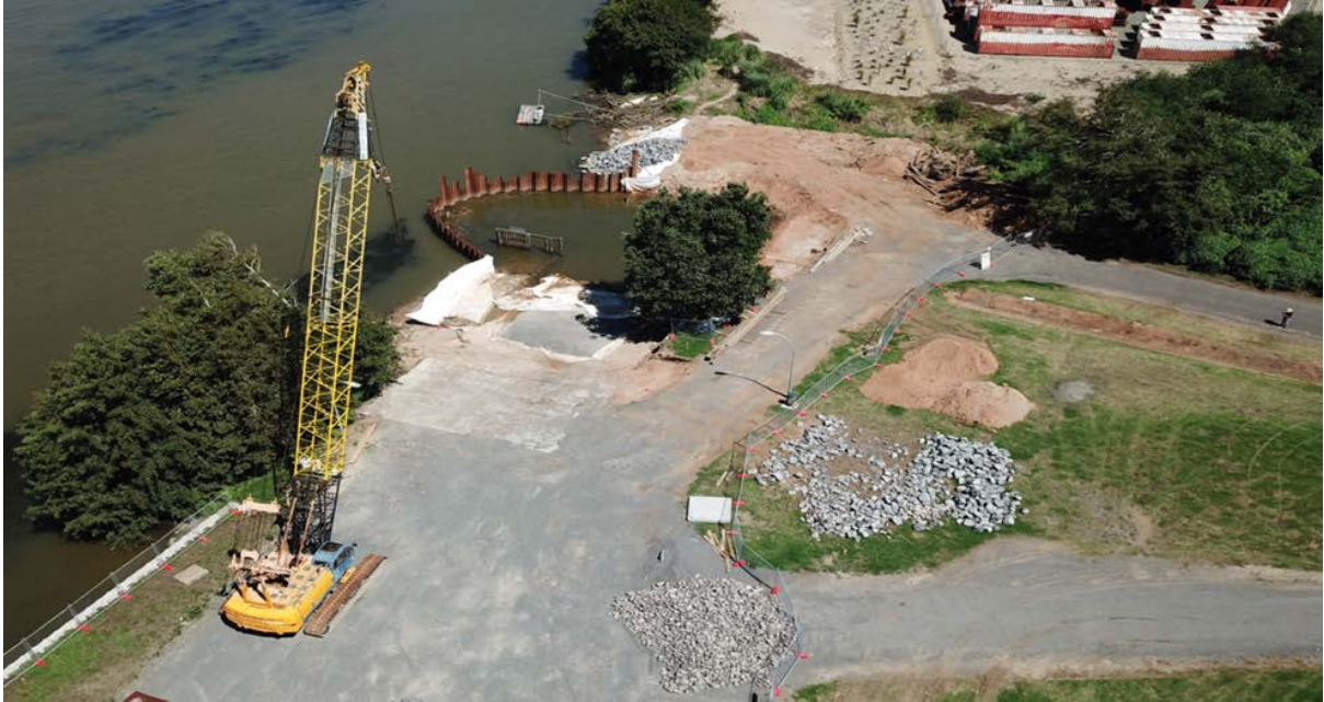
Elbow Boat Ramp Upgrade
