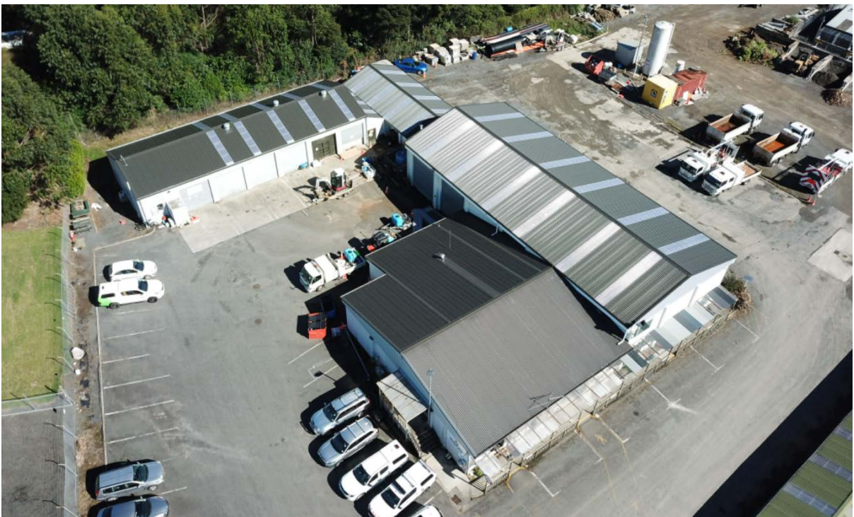
Brownlee Avenue Buildings Roof Replacements - Ngaruawahia
