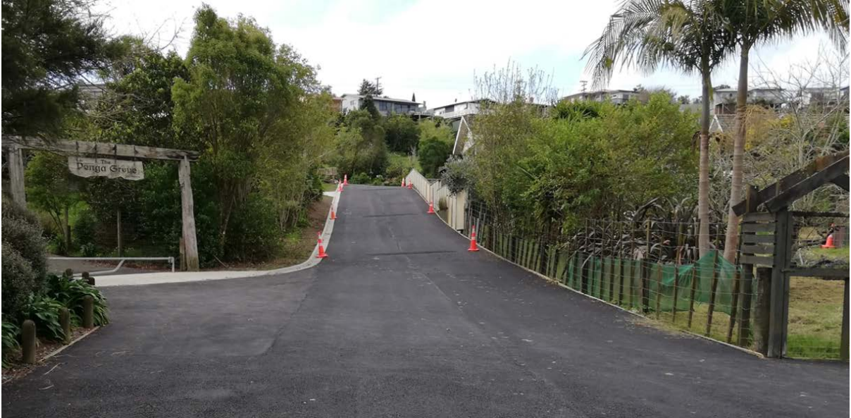
Green Cathedral Carpark Upgrade - Huntly
