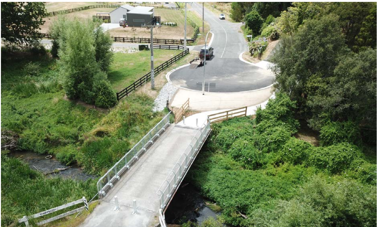
Annebrook Road Upgrade and Connection to Matangi Rd - Matangi
