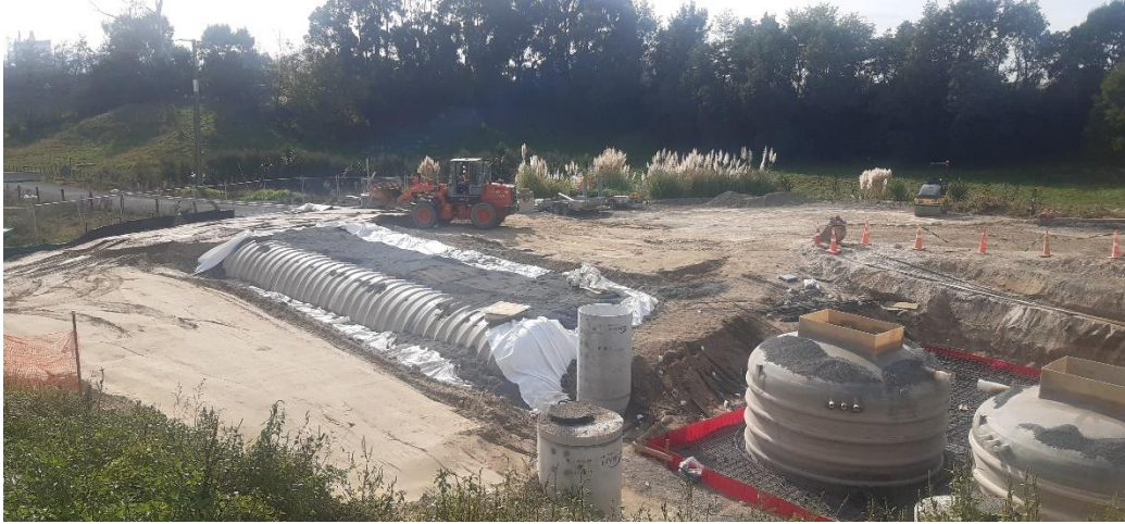
POAL WWPS - Earthworks are underway to form the finished ground level
