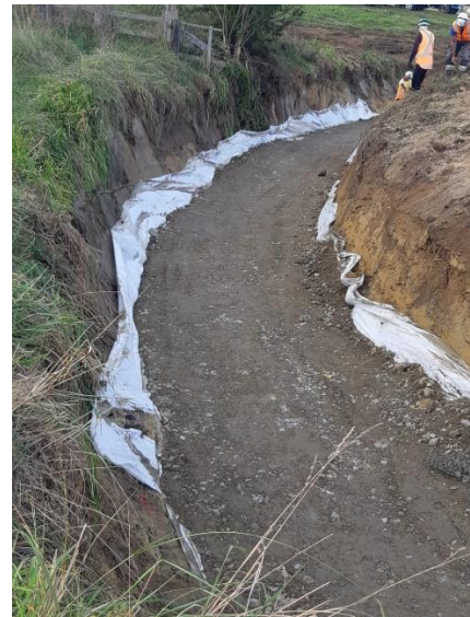
Filling Of Exist. Stream
