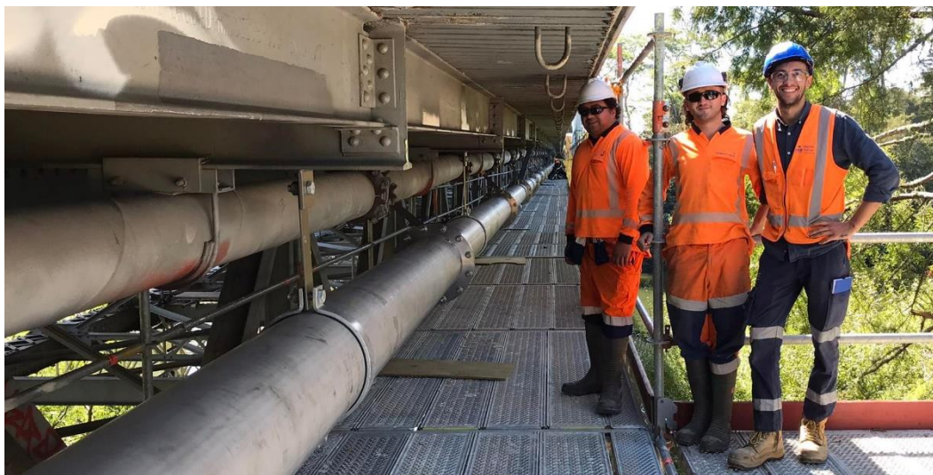
Ngāruawāhia Pipeline: Pipeline inspection and pressure test
