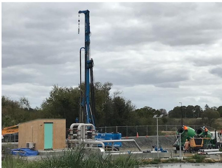
Piling for the MABR platform in progress.
