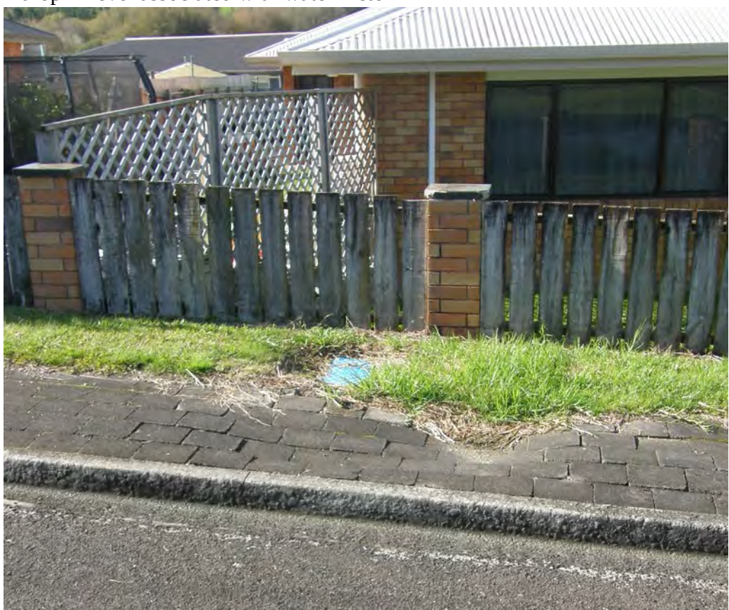
10) Outside #2 drop in level associated with water meter
