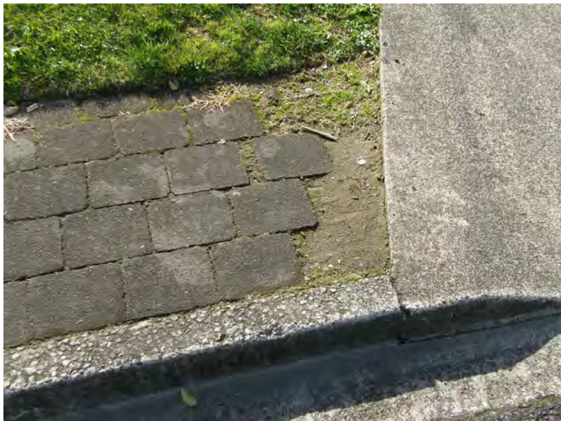
13) Missing section driveway interface at # 14. Only one side of the driveway
