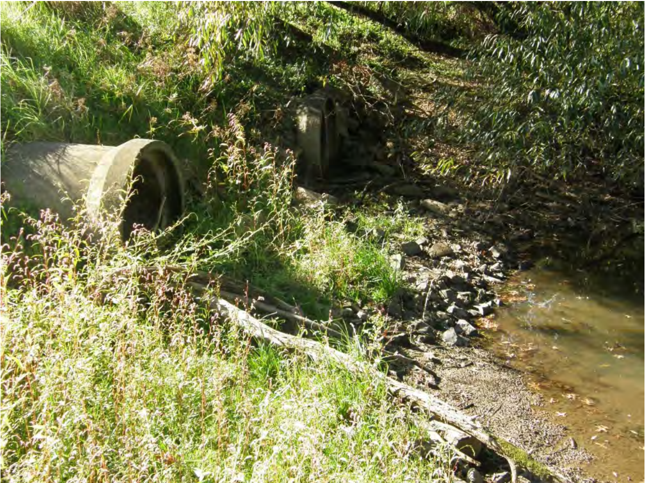
Culverts high above the water level. This is the inlet side.
