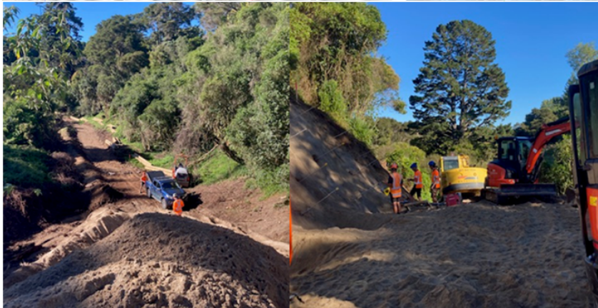
Managaonua Gully cycleway
