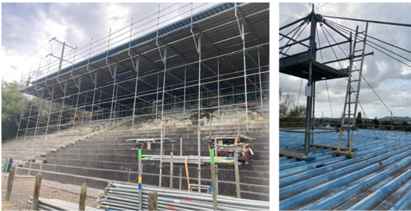
Huntly Grandstand roof replacement project
