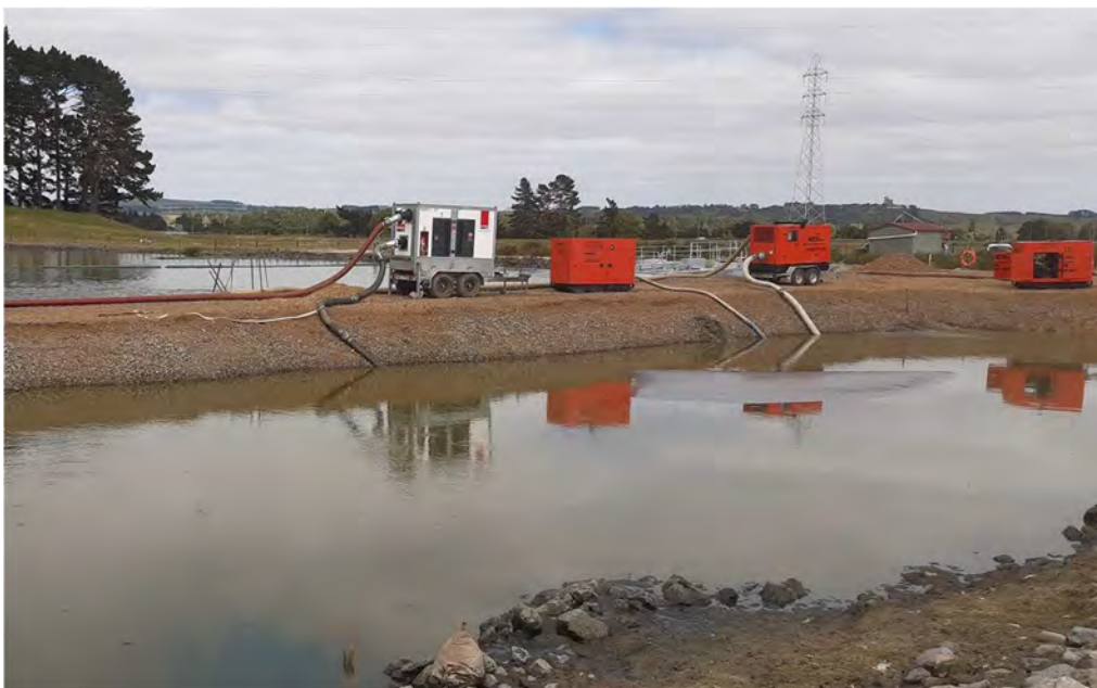
Meremere WWTP – reclamation works
