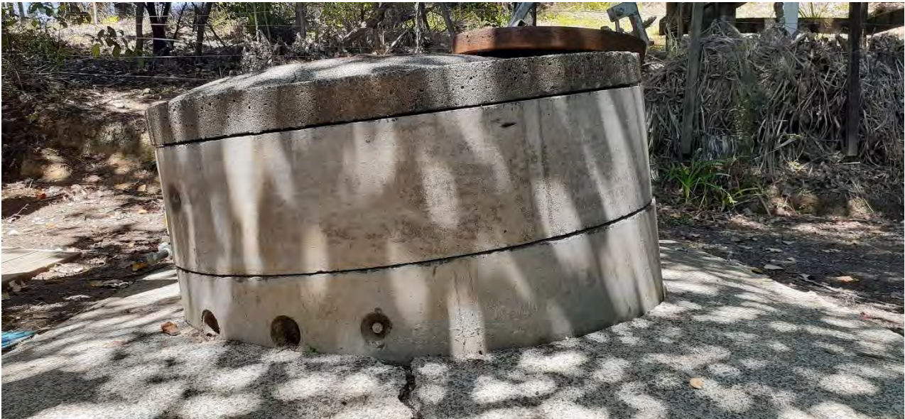
Figure 1 Te Akau Borehead
