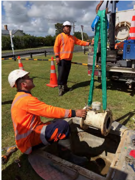
Old Magflow being removed from chamber – Bow St Reservoir
