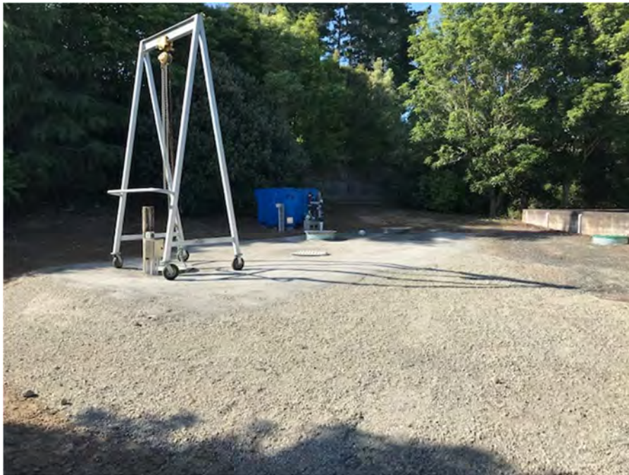
Te Kowhai WWTP post ground improvements
