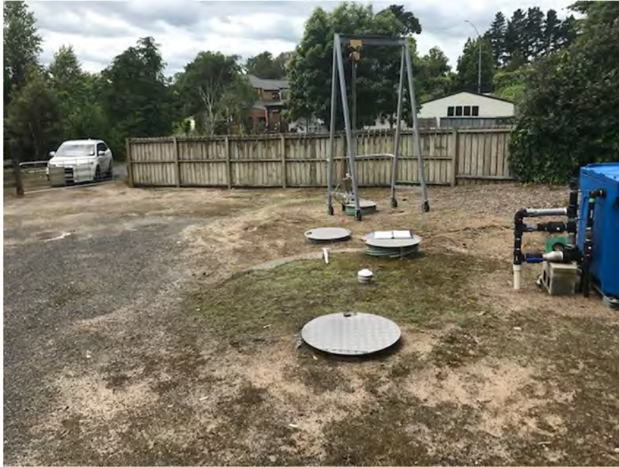
Figure 2 Te Kowhai WWTP pre ground improvements
