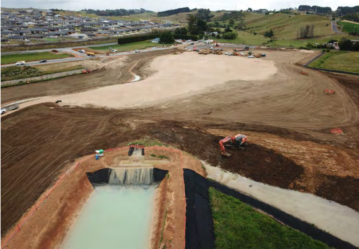
Drone image 22 December 2020 of desilting pond and topsoiling of surface underway.
