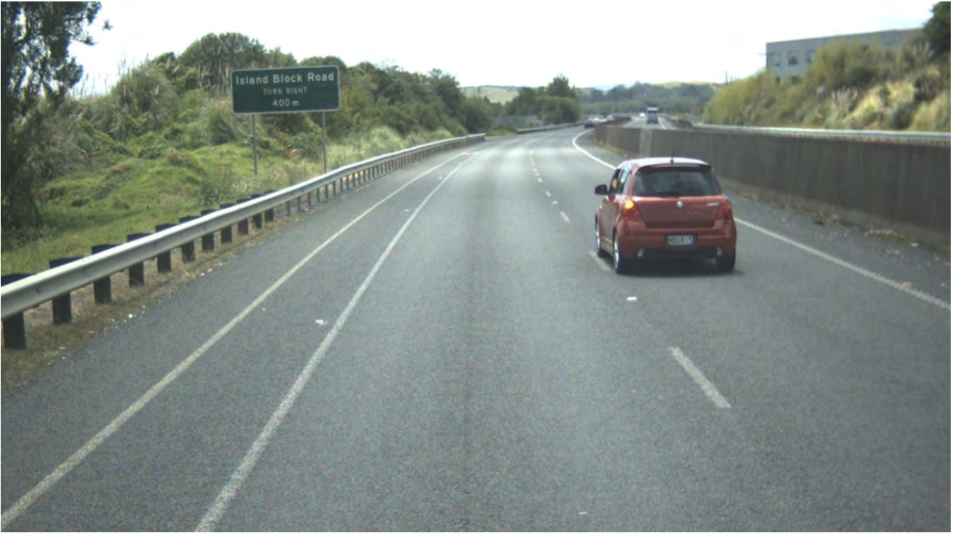
Figure 6: View looking north along SH1 showing advance warning signage for The Intersection
