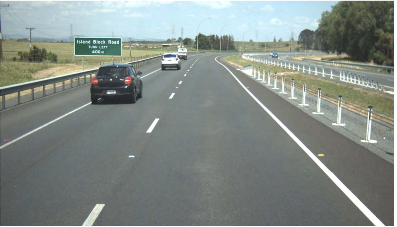
Figure 8: View looking south along SH1 showing advance warning signage for The Intersection
