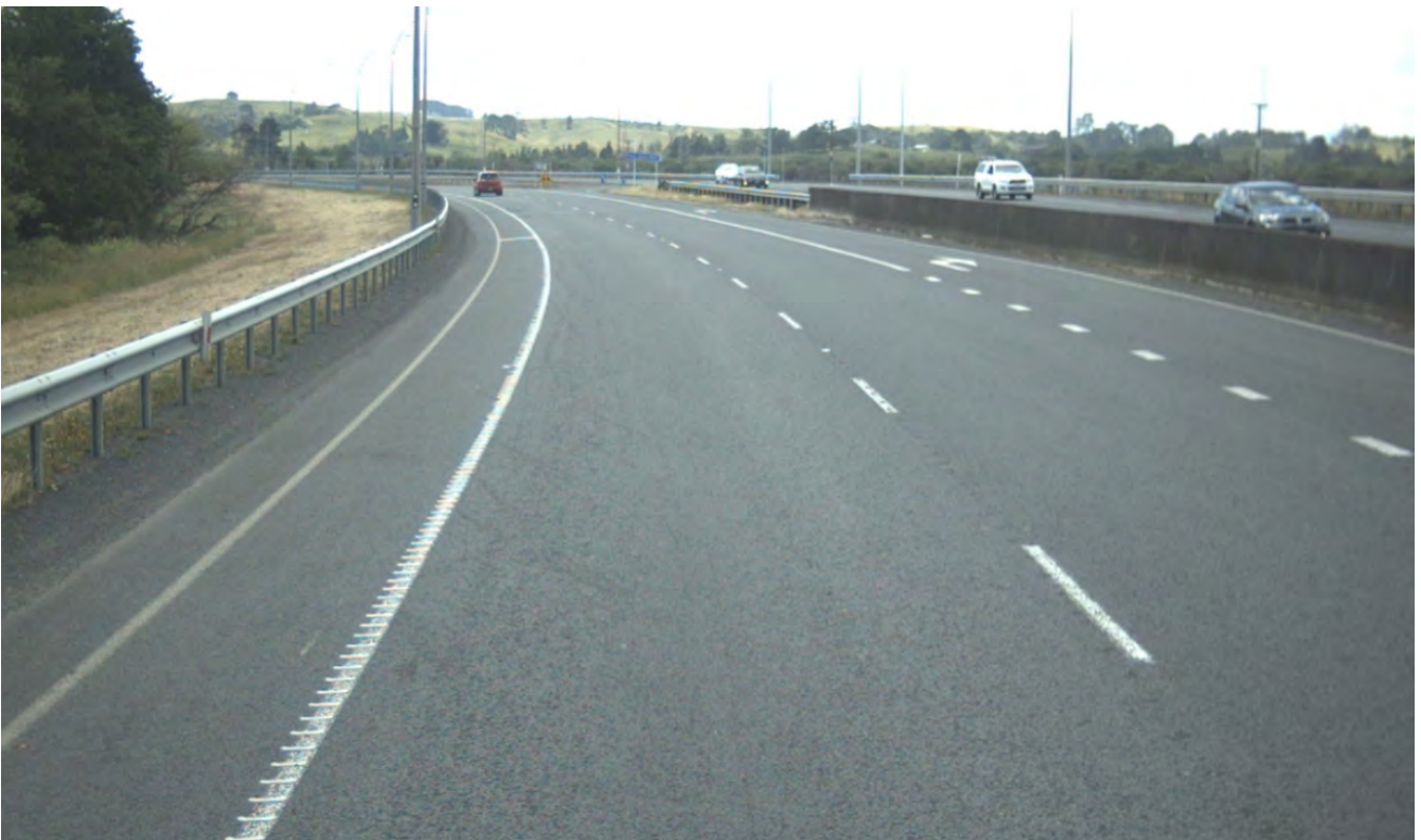
Figure 7: View looking north along SH1 showing the right turn bay and IDS signage at The Intersection
