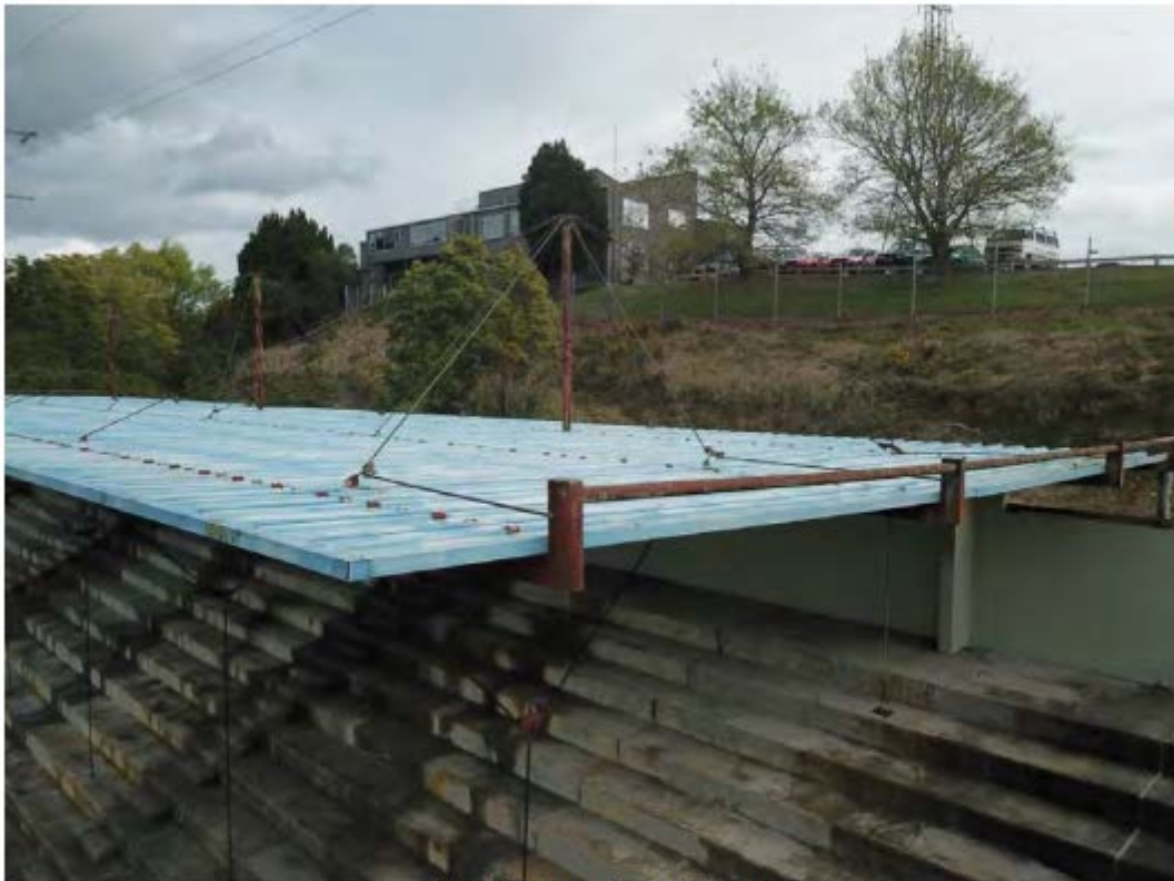
Huntly Grandstand Roof
