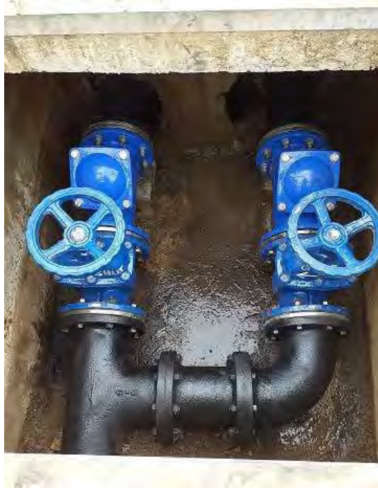
Rosser St PS non-returns and pipework completed.
