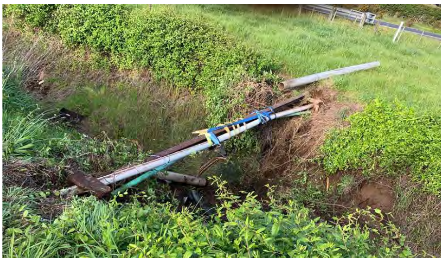
Temporary repair on 80mm water main
