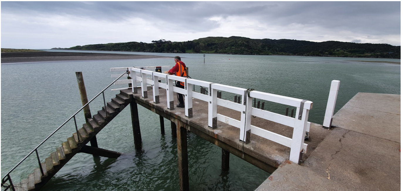
New handrails with stainless support brackets at Cliff St Jetty, Raglan
