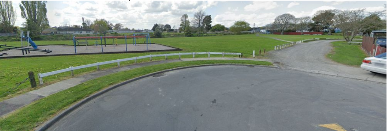
Harris Street, North end of bridge over Waahi stream
