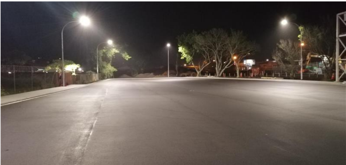
Asphalt surfacing in the car park well underway
