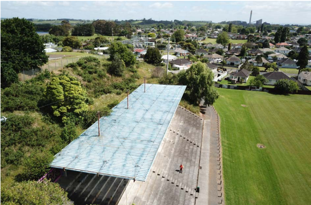
Huntly Granstand – Transpower transmission cables span the park above the grandstand roof
