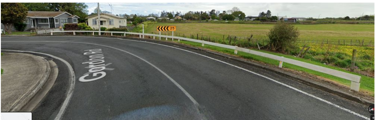
Gordon Road corner with Hakanoa Street
