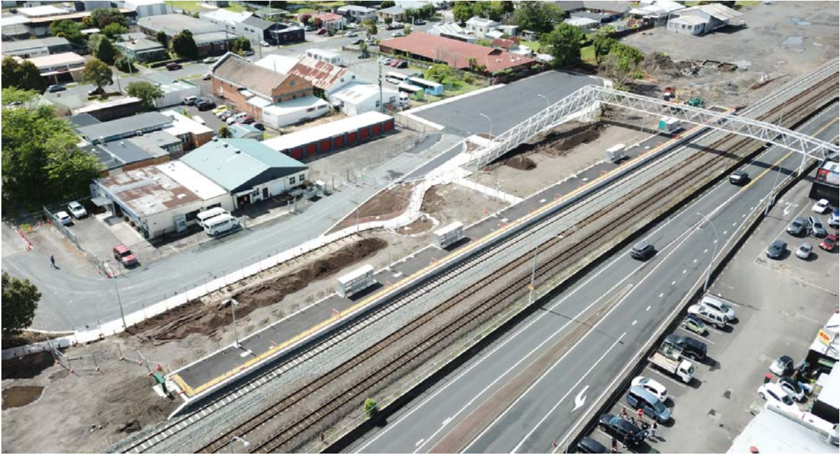
Aerial view of the railway platform and Park and Ride
