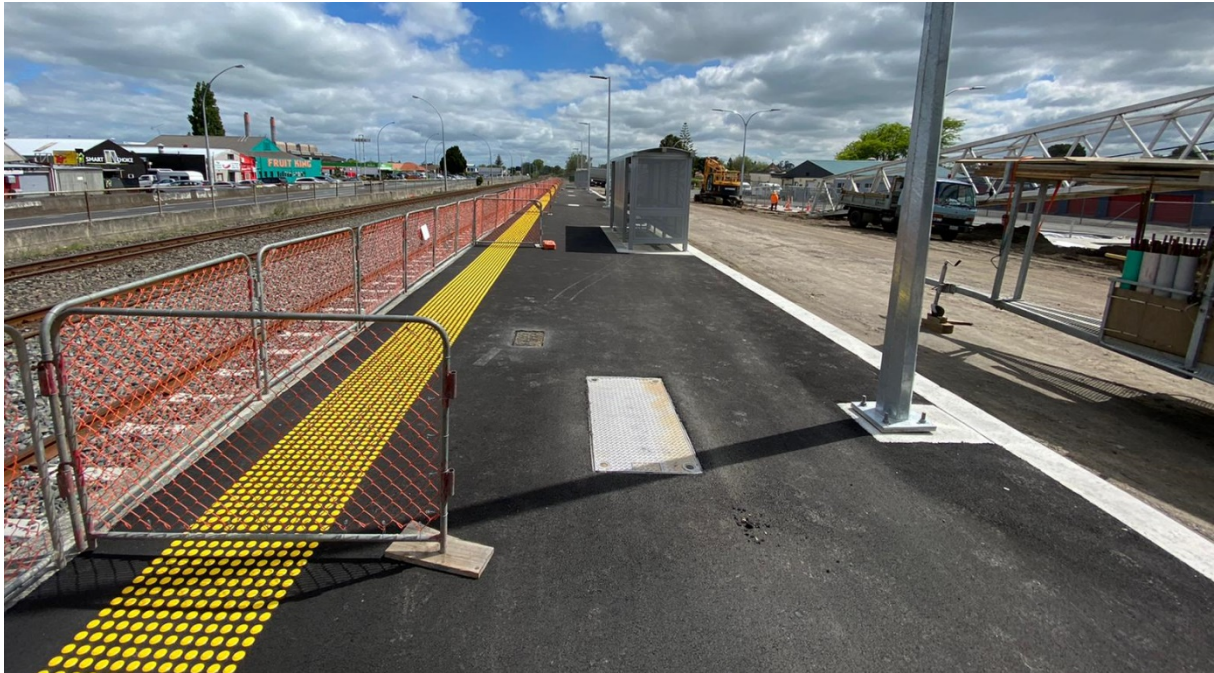
Completed railway platform
