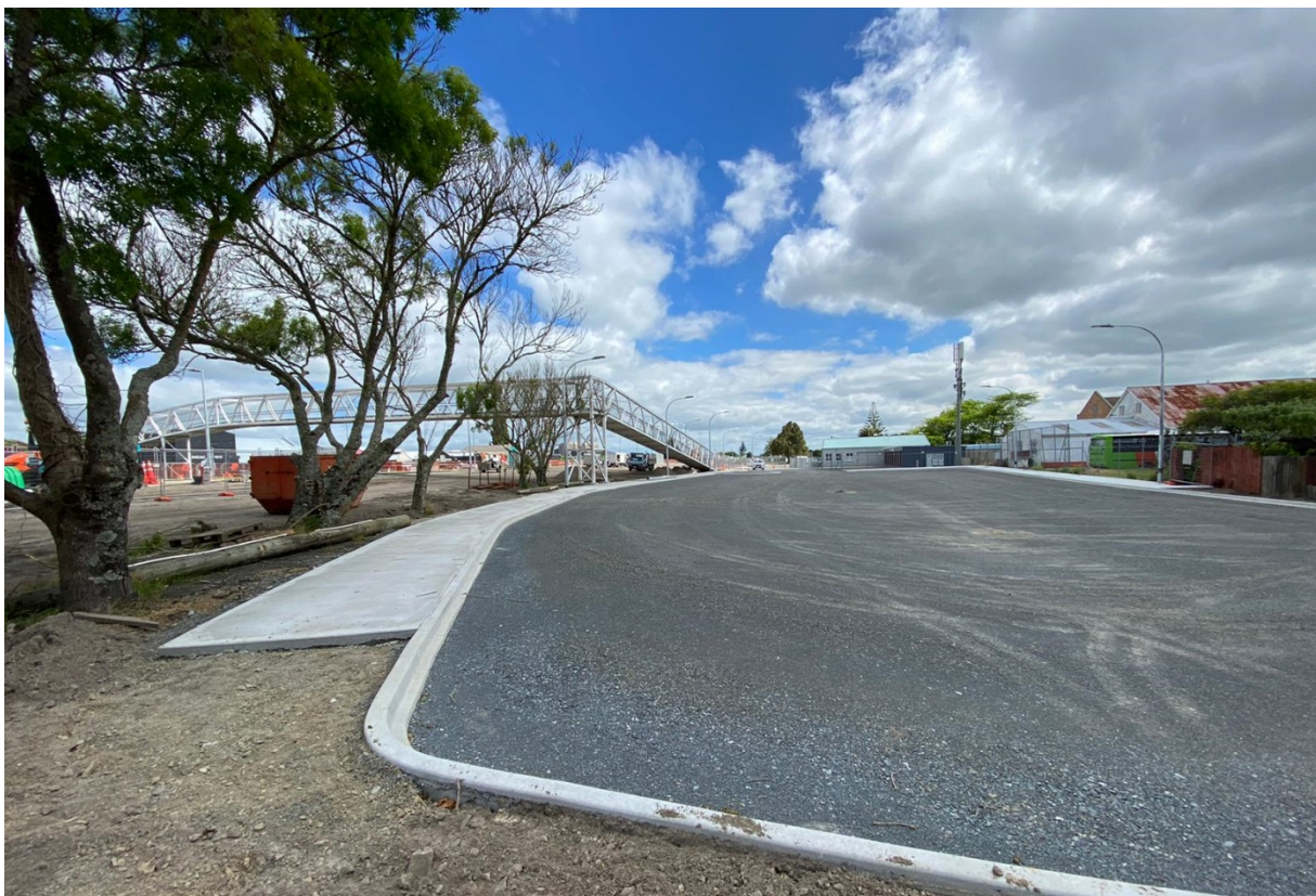
Park and Ride pavement nearing completion
