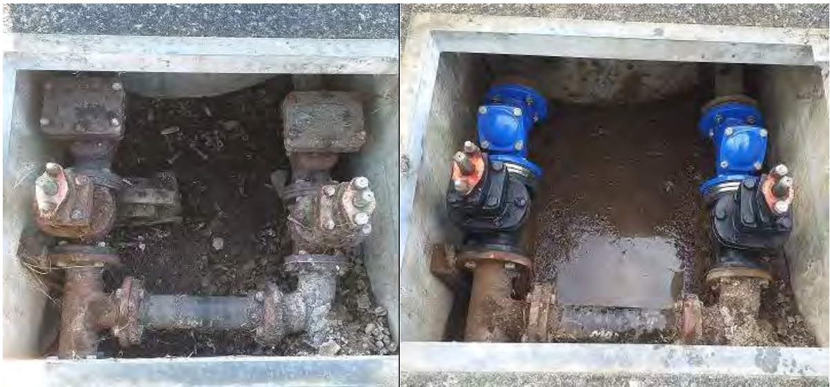
Images showing before and after renewal works at Stirling PI PS
