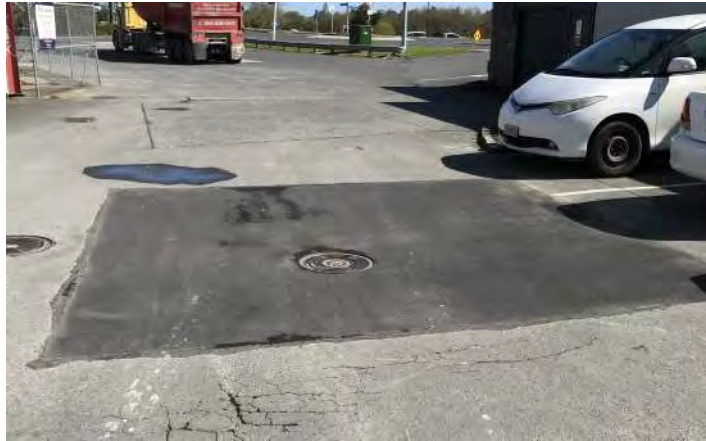
Reinstatement works completed with hot mix seal.
