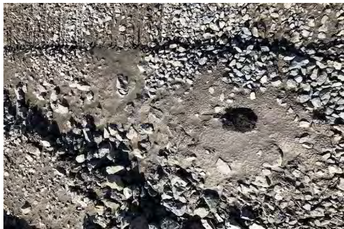
Te Kauwhata WWTP rock filter refurbishment
