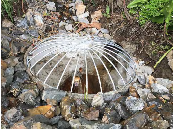
Image of the completed scruffy dome work at 3 Cross St, Raglan
