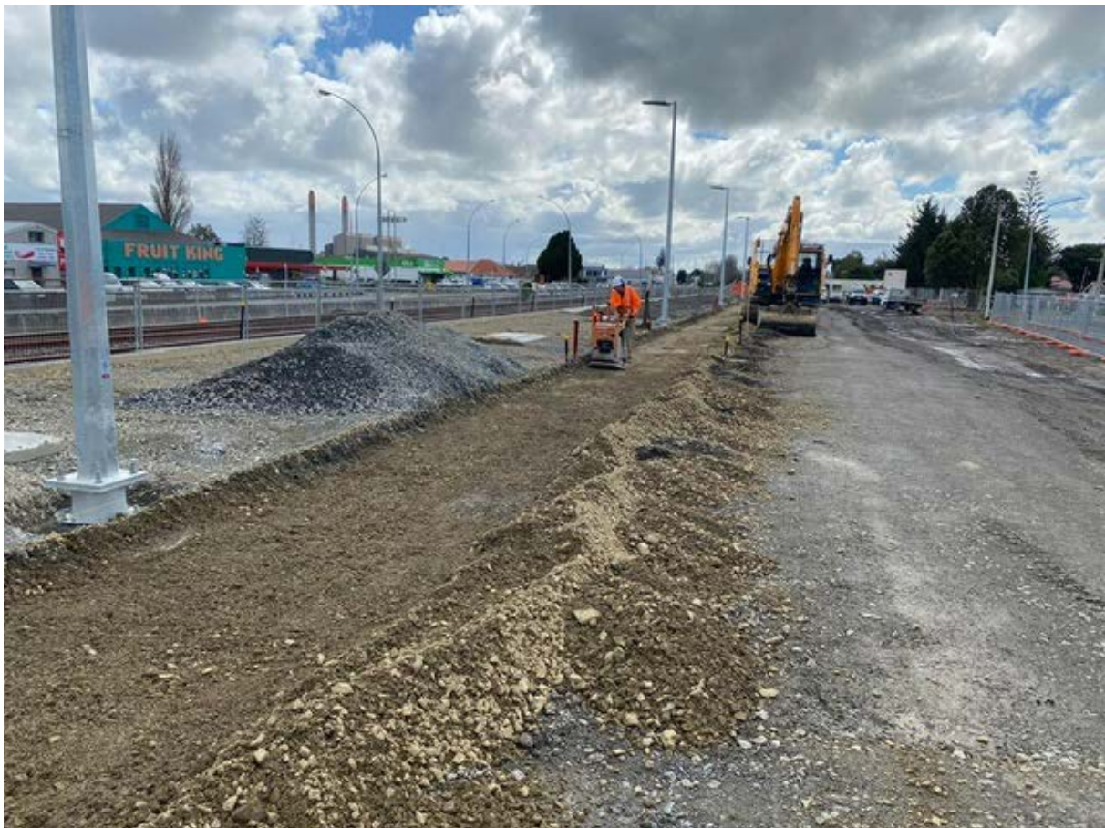
Preparations for the platform back concrete nib and fence
