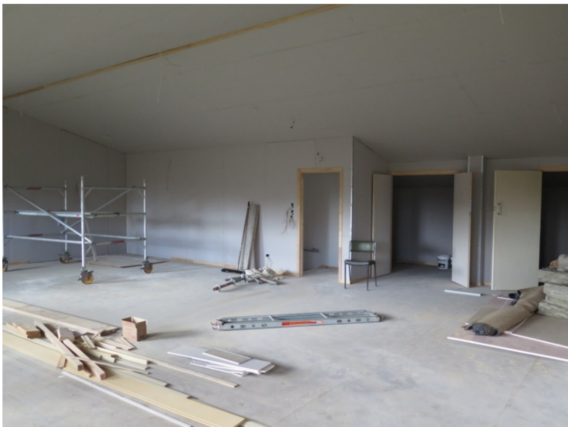
Community Room in Creative Space building with plasterboard up ready for plastering
