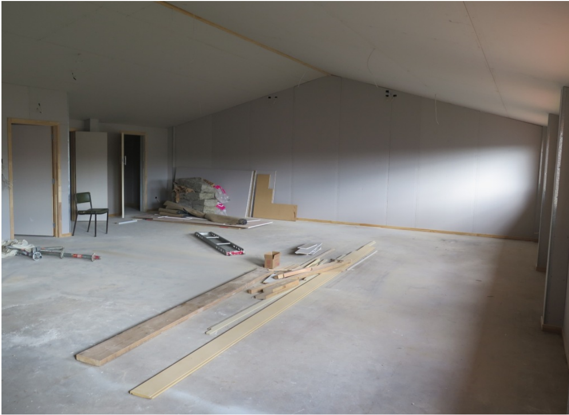
Community Room in Creative Space building with plasterboard up ready for plastering
