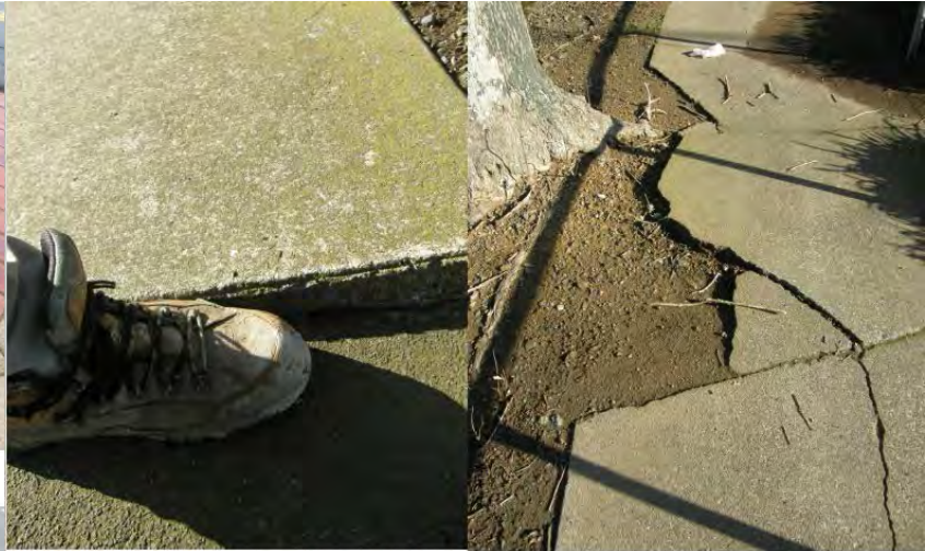
One week ago above, below is temporary fix until concreting job is scheduled in
