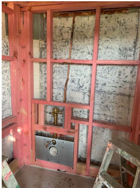
The Point, Ngaruawahia toilet refurbishment
