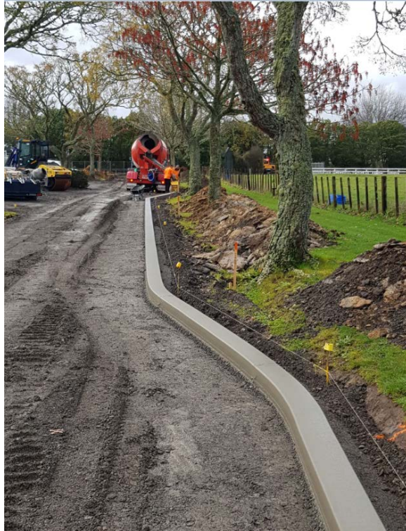
Kerbing underway at Jackson Street Cemetery
