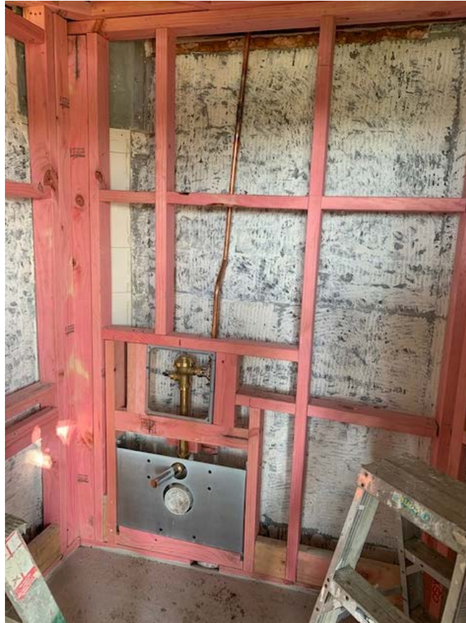
The Point Ngaruawahia toilet refurbishment
