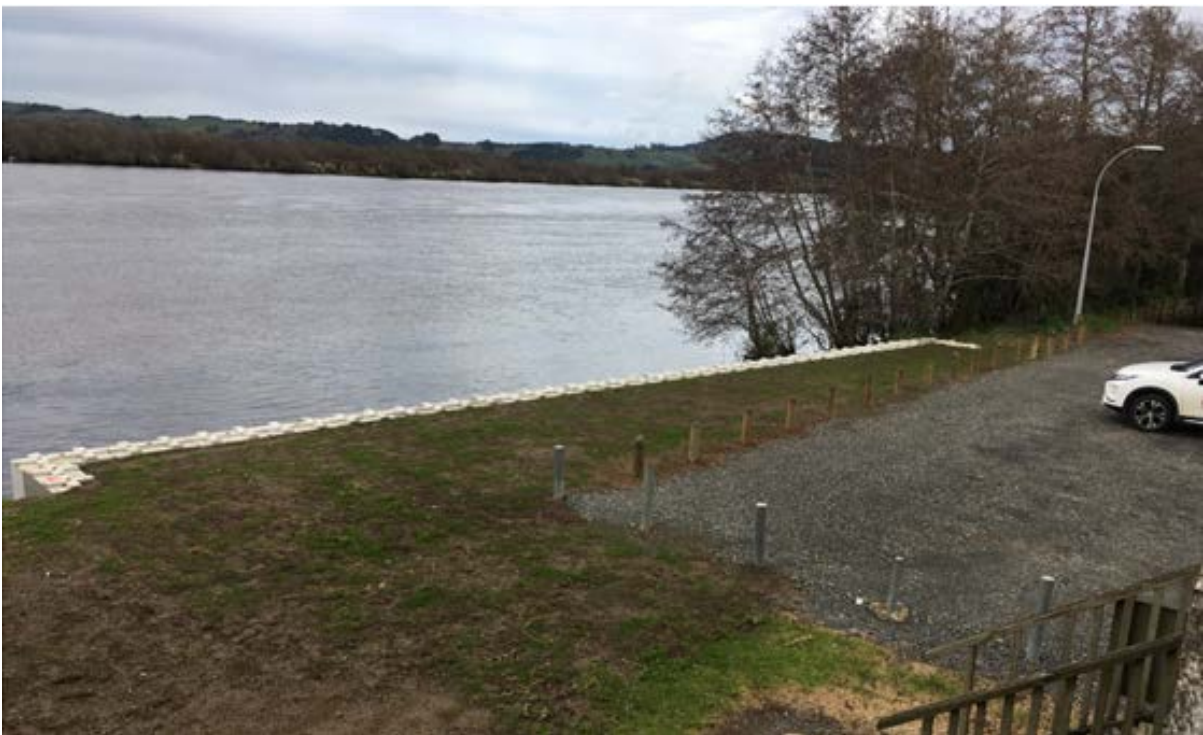
Completed erosion repair
