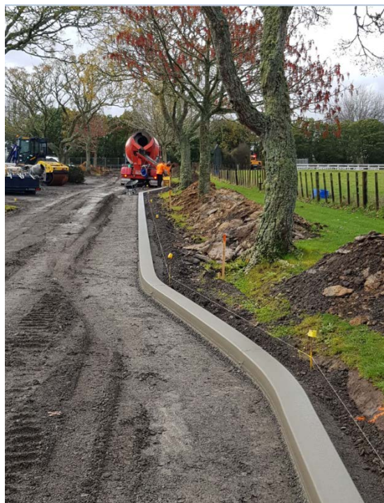
Kerbing underway at Jackson St Cemetery
