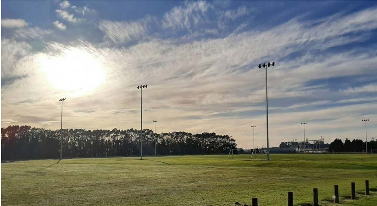
Completed sports field lighting
