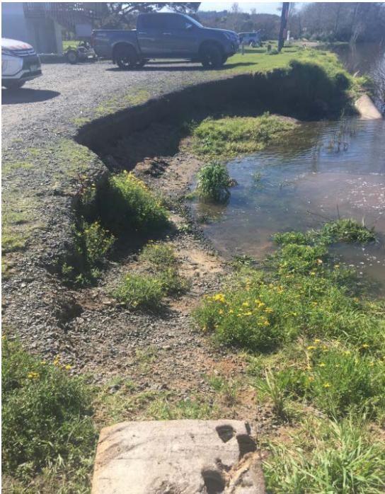
Riverbank erosion adjacent to boat ramp before repair
