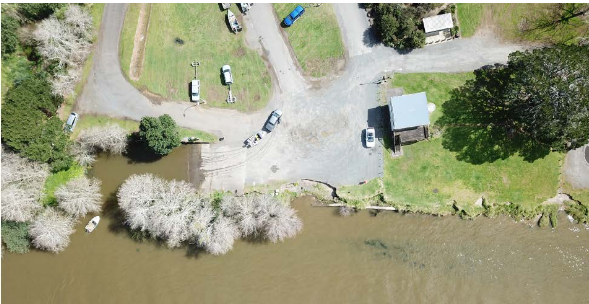
Riverbank erosion adjacent to boat ramp before repair
