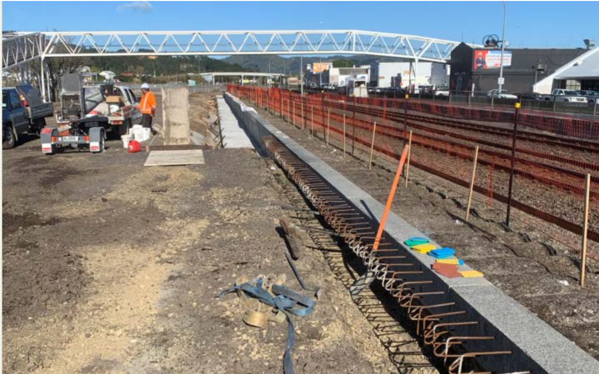
Installing new panels to raise the height of existing section of the platform to meet new standards
