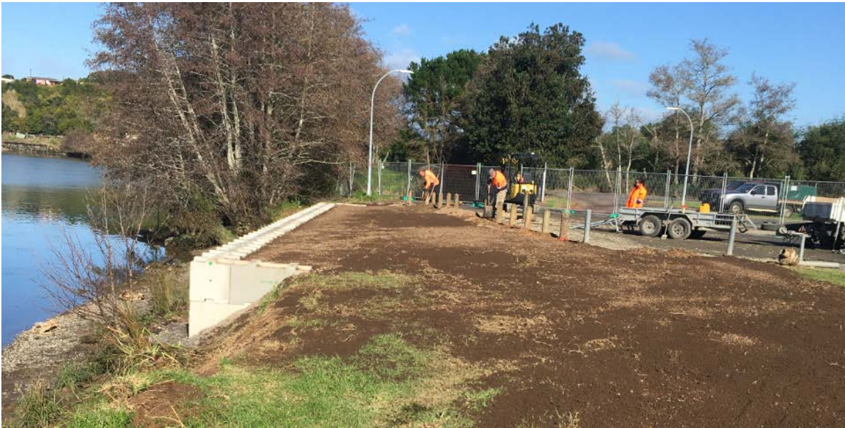
Completed erosion repair
