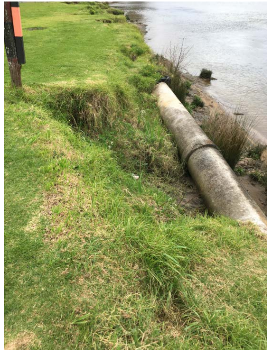
Riverbank erosion adjacent to boat ramp before repair
