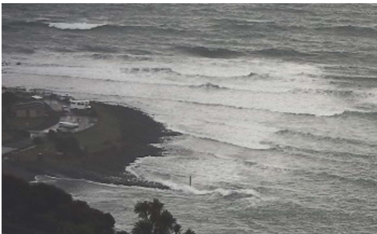
Figure 1.1. Over-topping of the Manu Bay breakwater in mid-2019; monitoring image.
