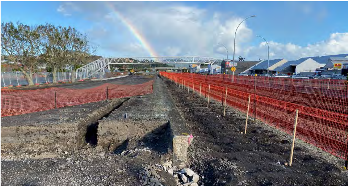
North end of the railway platform looking south
