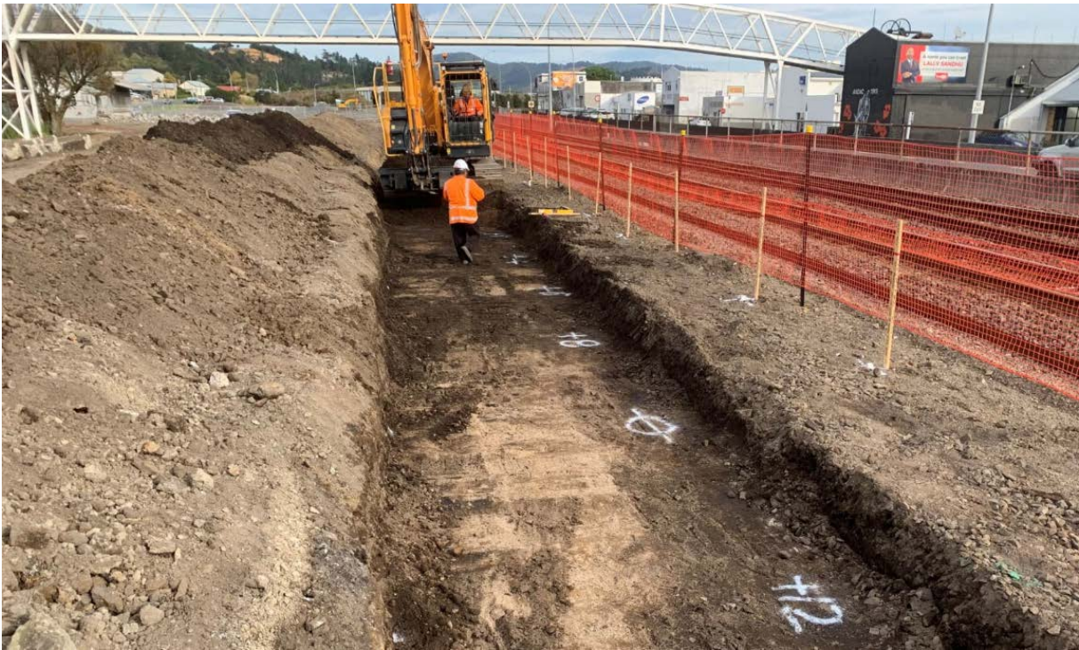
Foundation cut along front of existing platform
