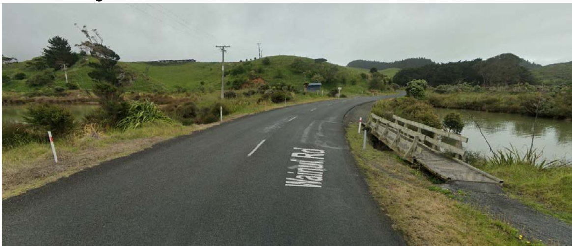
Walkway Bridge opposite Wastewater Treatment Plant
