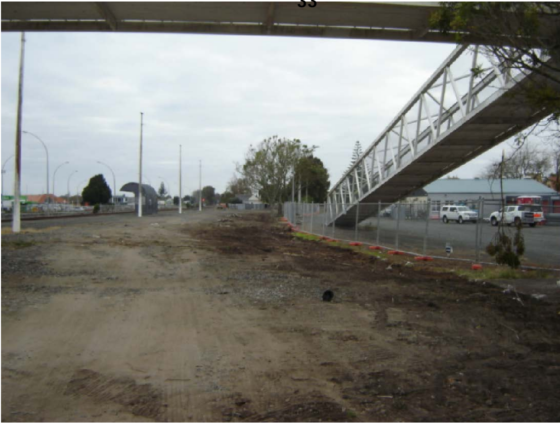
Site cleared ready for construction to get underway
