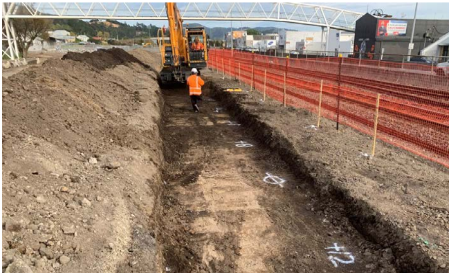
Foundation cut along front of existing platform
