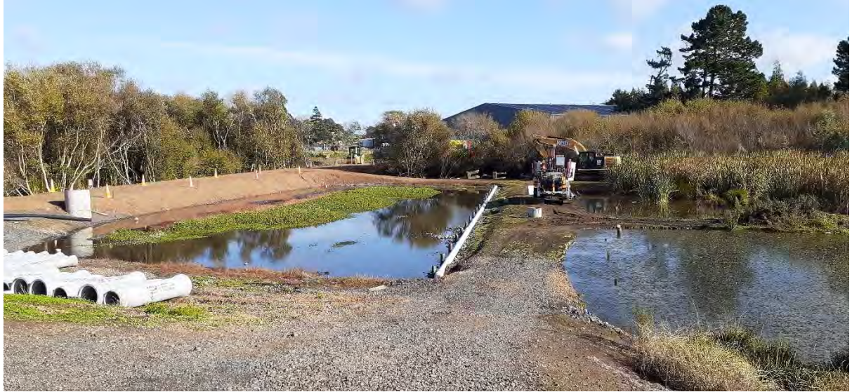
Geotechnical investigation at Te Kauwhata WWTP
