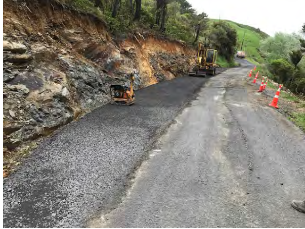
Wairamarama-Onewhero Road slip repair
