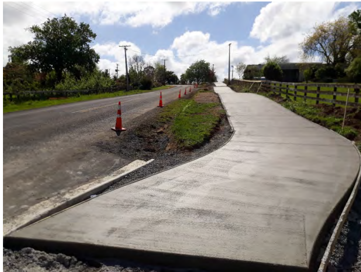
Travers Road Footpath Works
