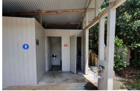
Women's side – additional pan & basin added
