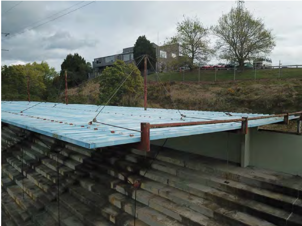
Huntly Grandstand Roof
