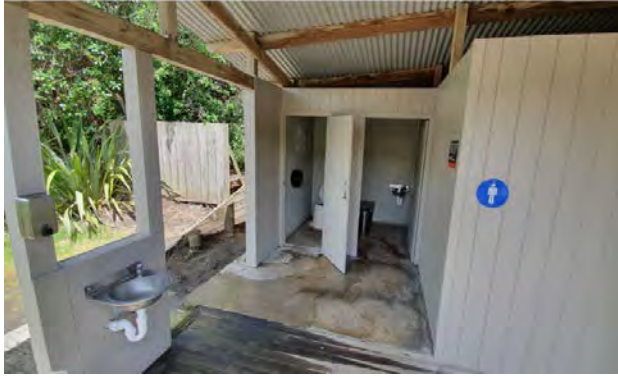
Men's side – additional pan & basin added
