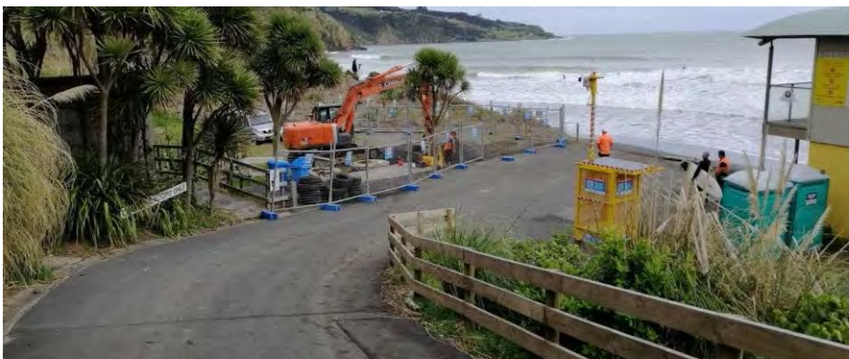
Progress photo of construction mobilised – 2 September 2019
