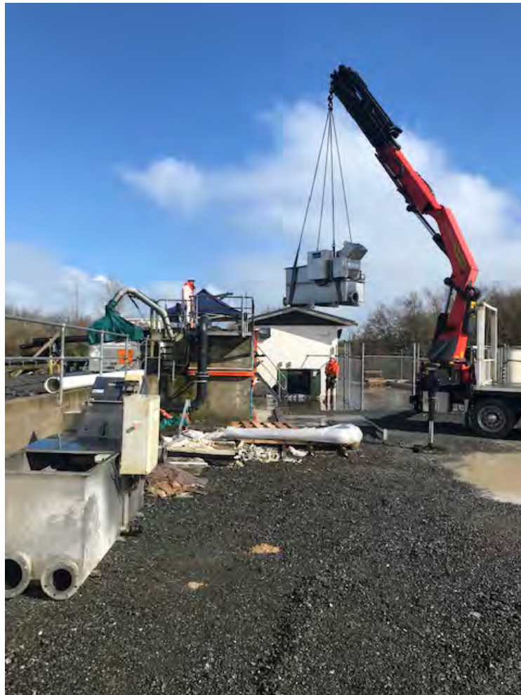
Step screen installation
