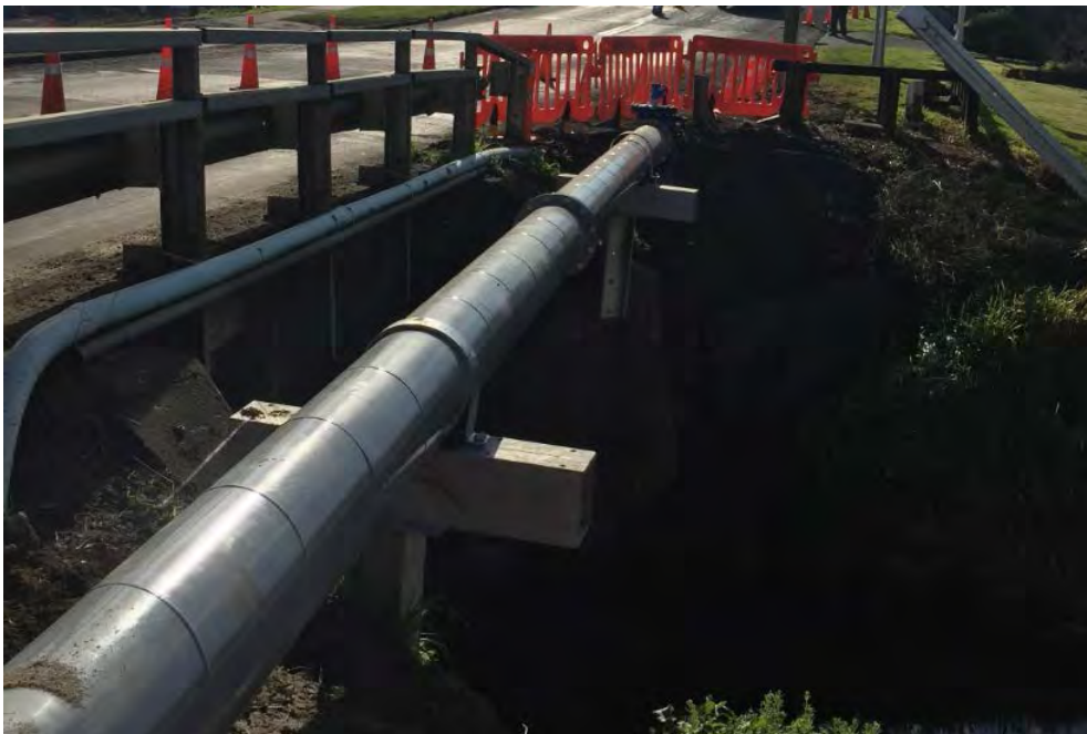
Tuakau Bulk Main Pipe Bridge
