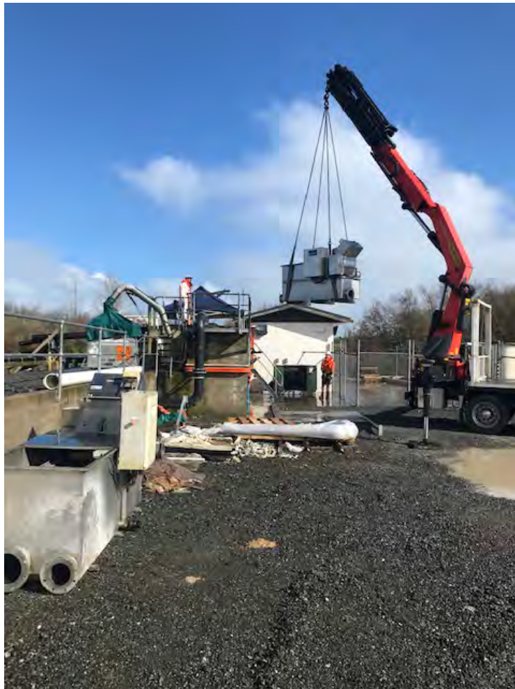
Step screen installation
