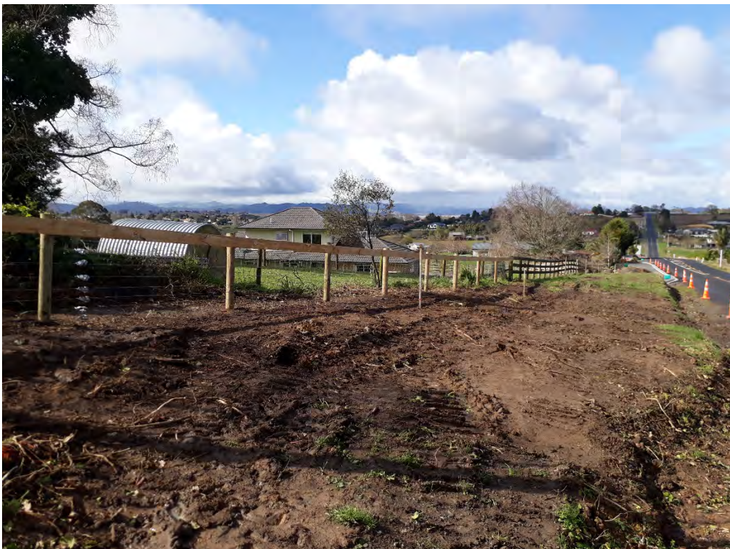
Progress Photo of fencing and formation works required immediate near Moorfield Rd – 23 August 2019
