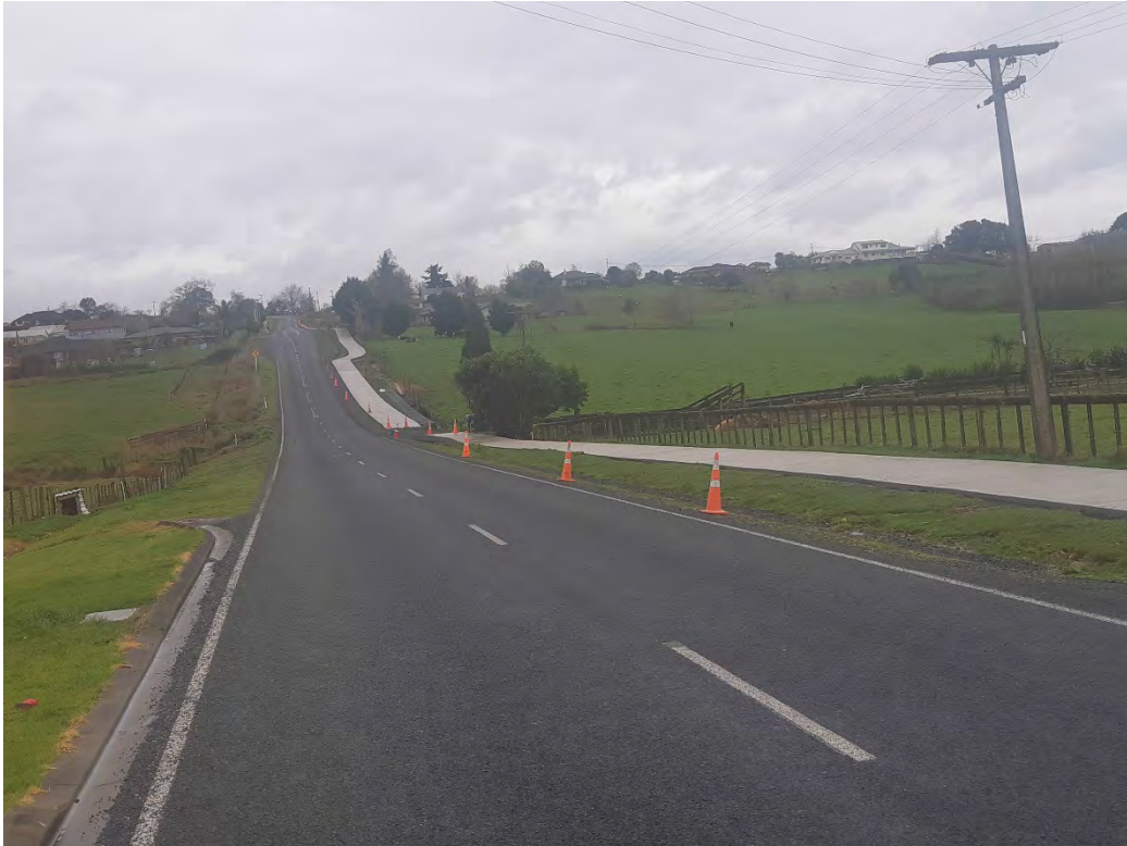
Progress Photo of Concrete constructed to date – 23 August 2019
