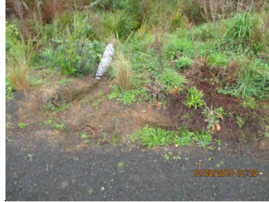
Drain within Lot 20
