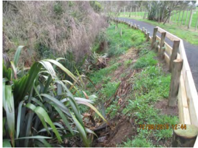
Repaired slip outside of Lot 20
