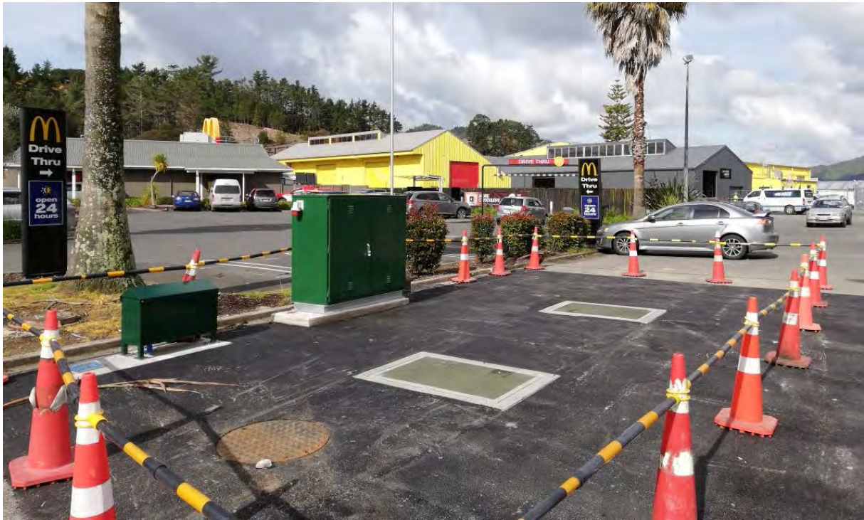
Works completed at the new pump station
