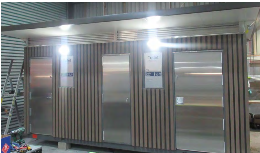
Exeloo making final touches to the St Stephens Toilet
