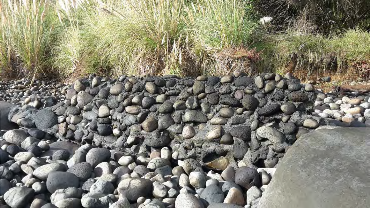
Existing rock wall erosion measure
