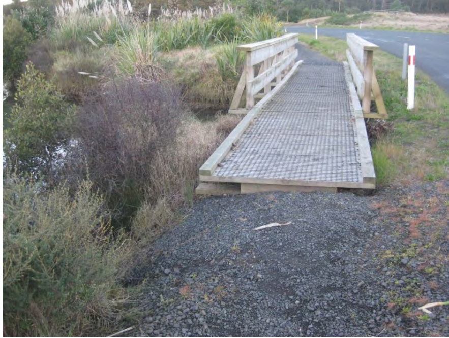
Wainui Road Footbridge
