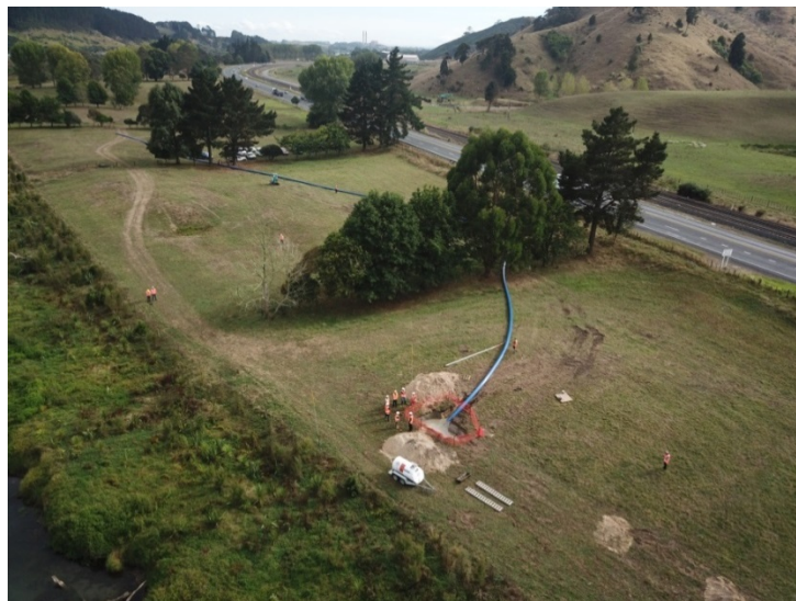
Drill rig on site for installing pipe under the Waikato River
