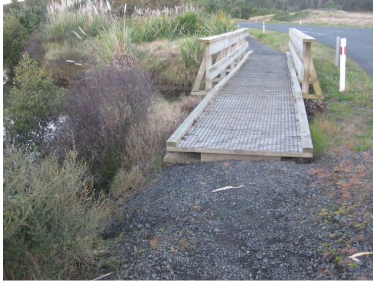
Wainui Road Footbridge
