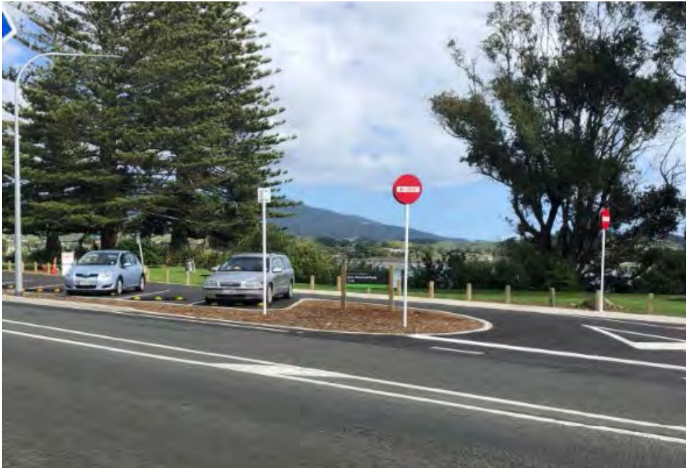
Joyce Petchell Park – Sign and Bollard Install Completed
