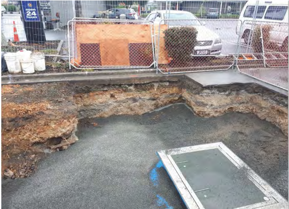
Pump Station works awaiting final reinstatement and WEL power supply
