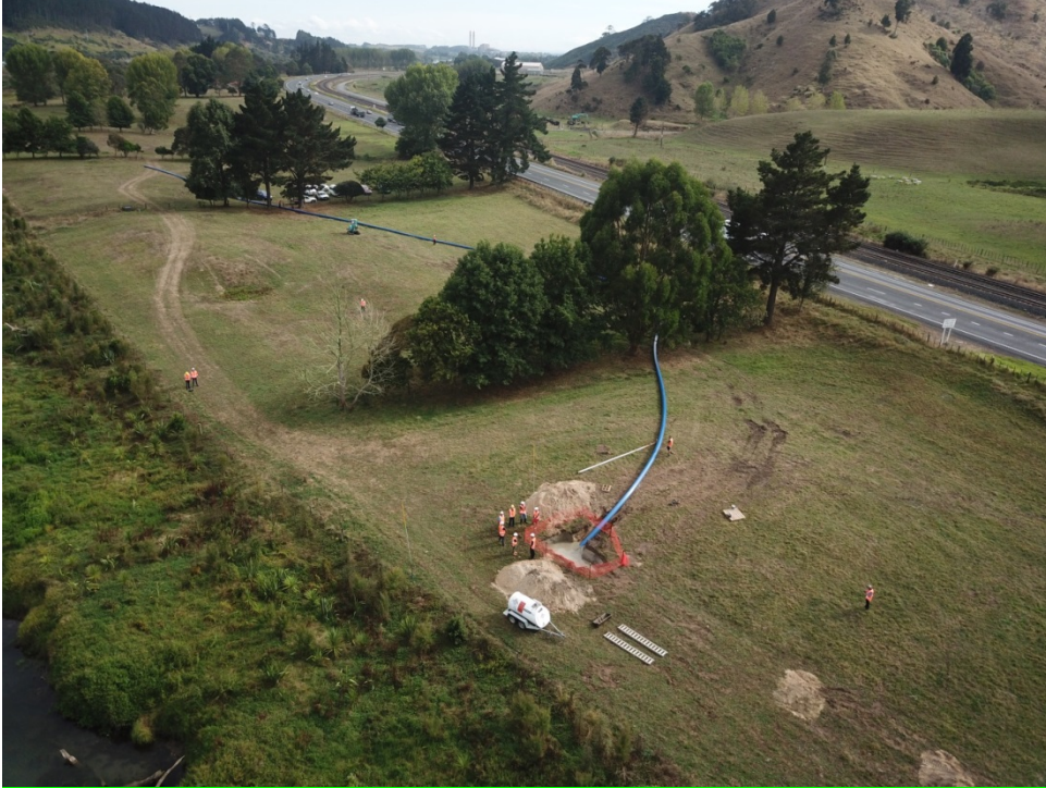
355mm PE Pipe being pulled under Waikato River
