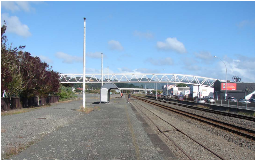
Existing Huntly railway platform
