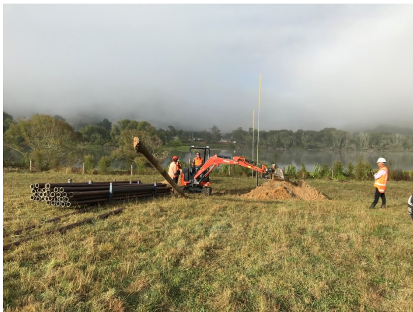
Drill Head emerging from River crossing on SH1 side
