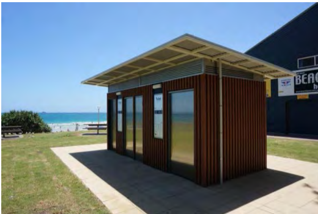
Example toilet block (note this is a 3 pan)
