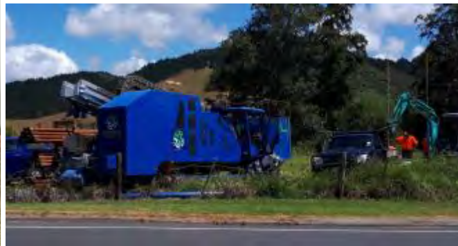
Drill rig on site for installing pipe under the Waikato River .
