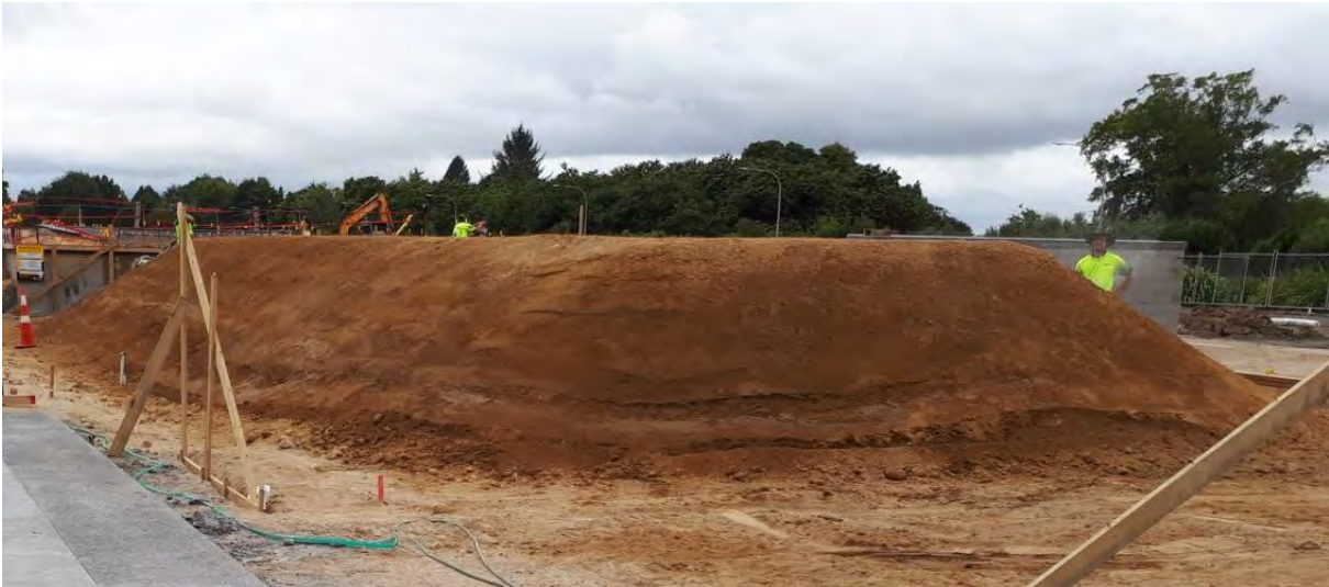
Formed earth mound for slides, rock climb holds, climb grips & ropes and inground trampolines.
