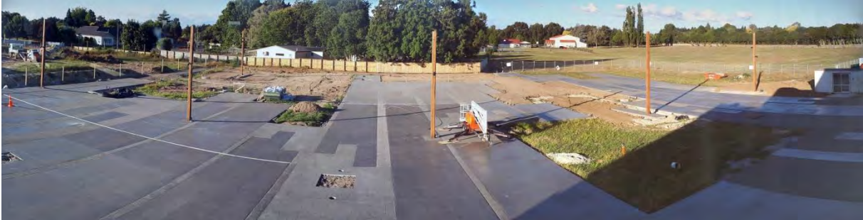
Piazza view from 1 st floor of commercial building Block C
