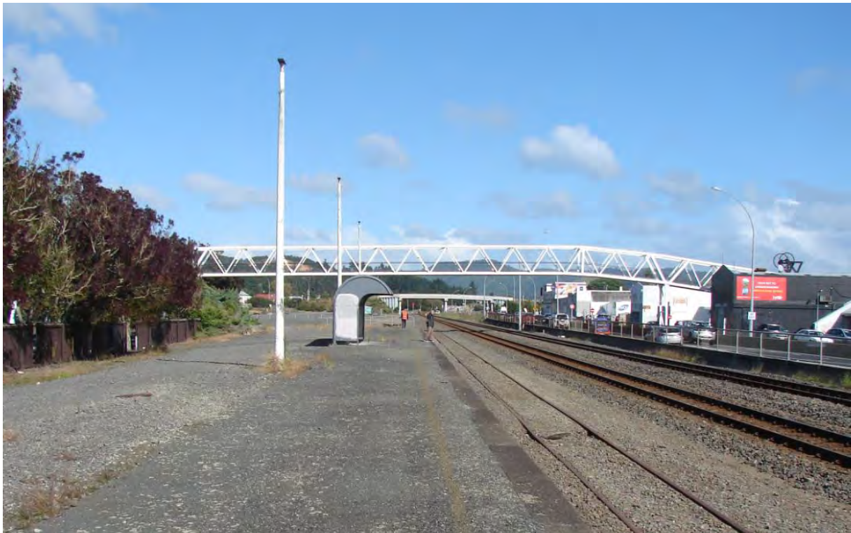
Existing Huntly railway platform
