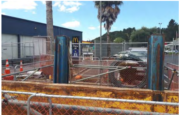
Shoring needed for built up worksite and soil conditions encountered
