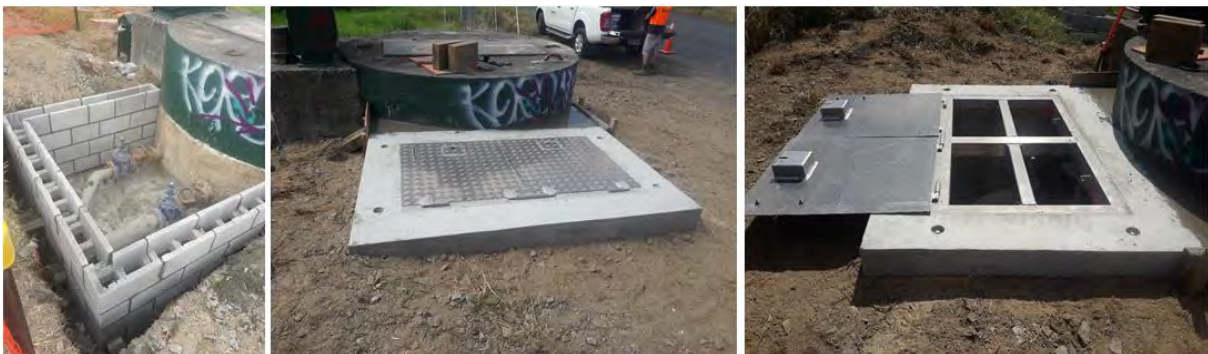
WDC wastewater pumpstation located on East Mine Road, Huntly – a full valve chamber build with additional RPZ (washdown) upgrade
