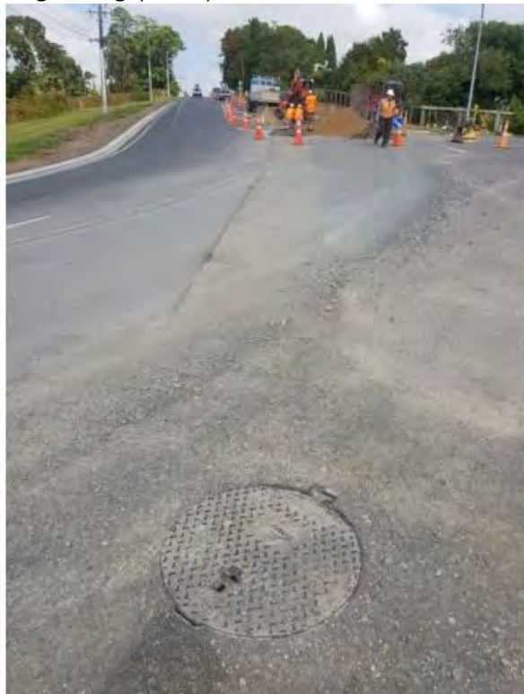
Site 1 - Te Kauwhata Rd wastewater upgrade works
