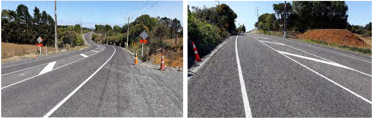
Whangarata Road completed rehabilitation
