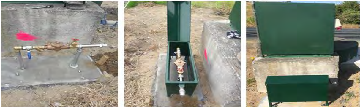
WDC wastewater pumpstation located on East Mine Road, Huntly – a full valve chamber build with additional RPZ (washdown) upgrade
