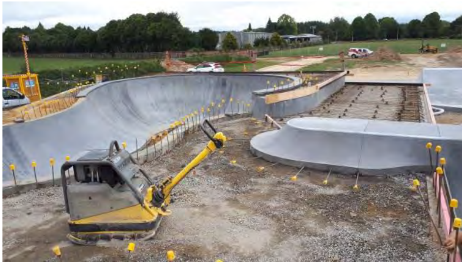
Skatepark pool bowl, double quarter pipe with table top, and drop-in ramp
