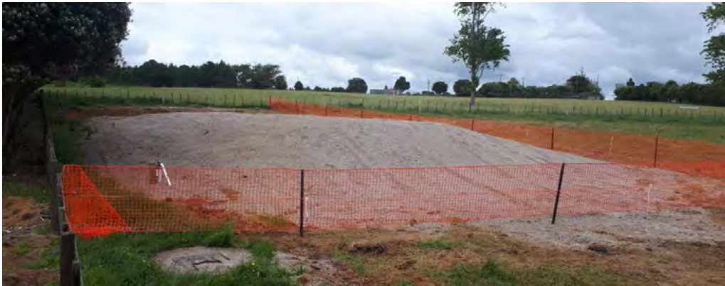
Wisconsin Mound for effluent soakage and evaporation
