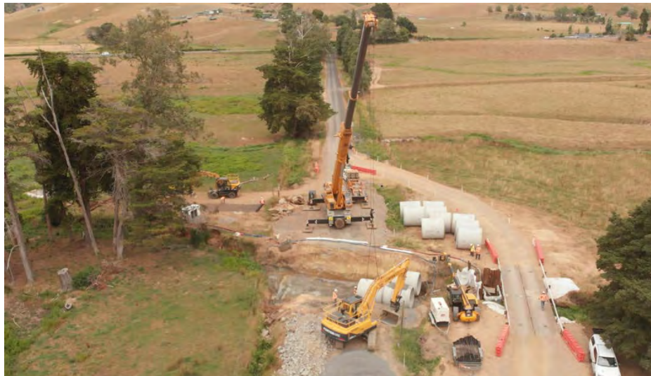
Dimmock Road Culvert Installation
