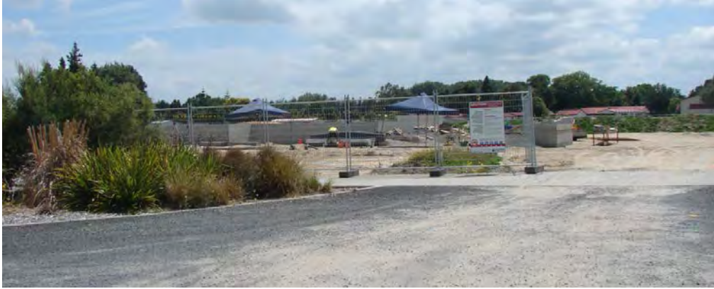
Skate Park retaining walls under construction.
