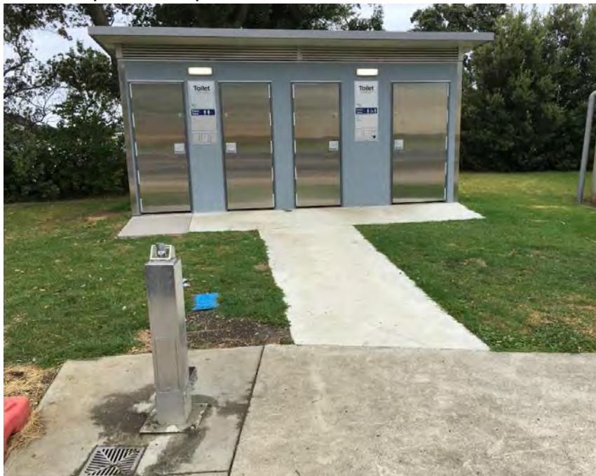
New toilet block opened on 2 November
