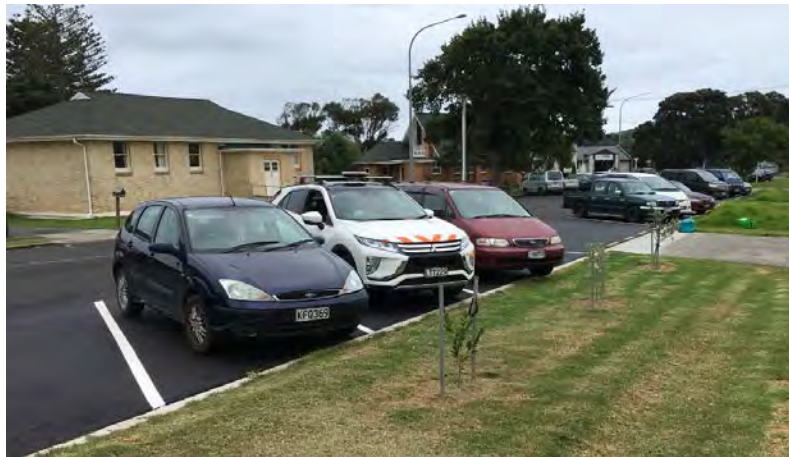
Completed Stewart Street Car Park
