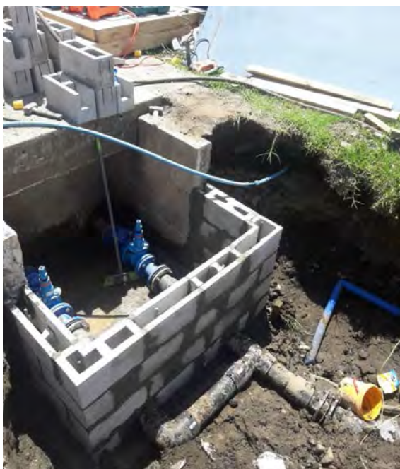
Valve chamber under construction
