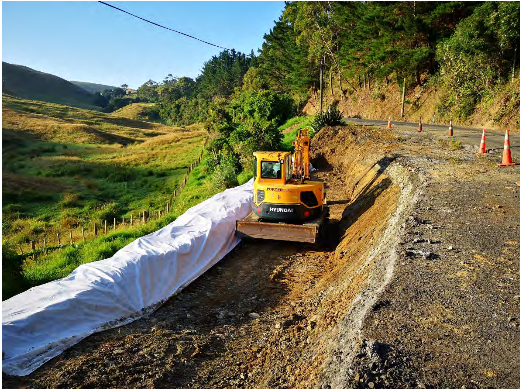
Slip repair work on Port Waikato – Waikaretu Road
