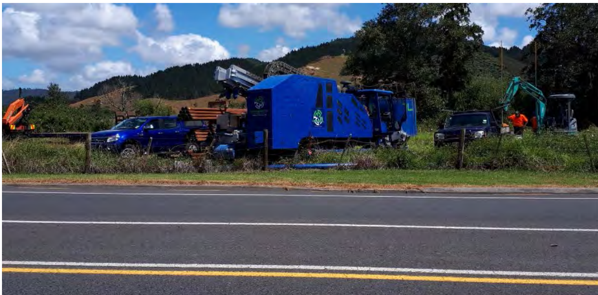
Drill rig on site
