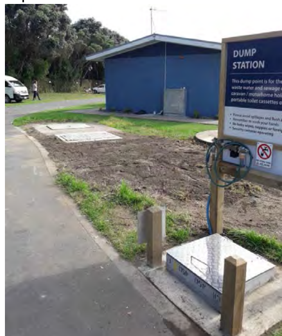
Completed camper blackwater dump station
