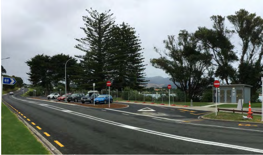
Completed Car Park and Toilet
