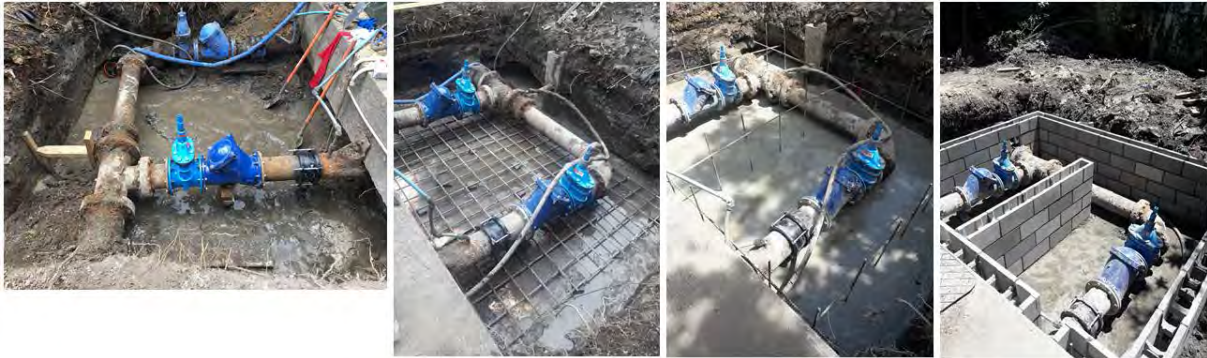
WDC wastewater pump station located within the grounds of Huntly Primary School – non-return valve and isolation valve replacement with a full valve chamber construction in progress
