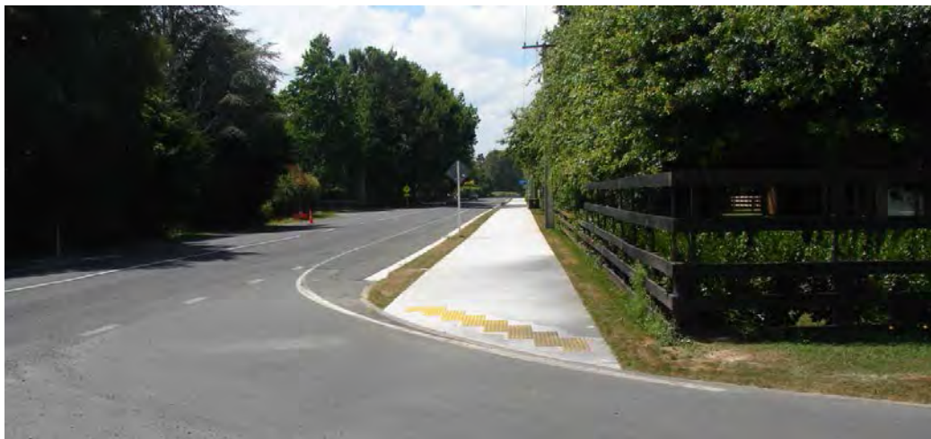
Tamahere Walkway/cycleway – part of the Te Awa Cycleway
