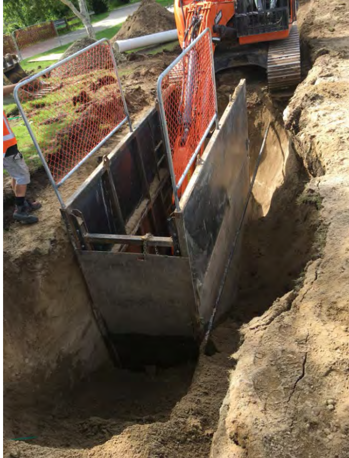
Trenching shield in use
