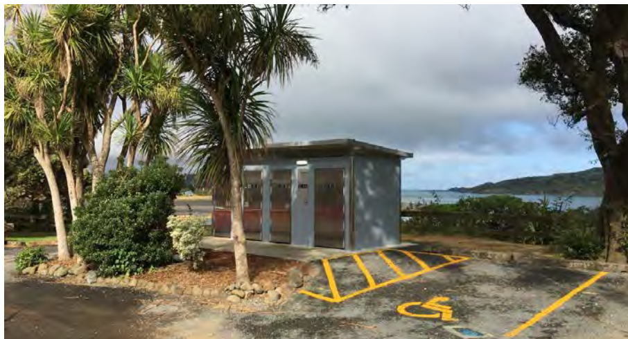
New Cliff Street Toilets opened on 20 December
