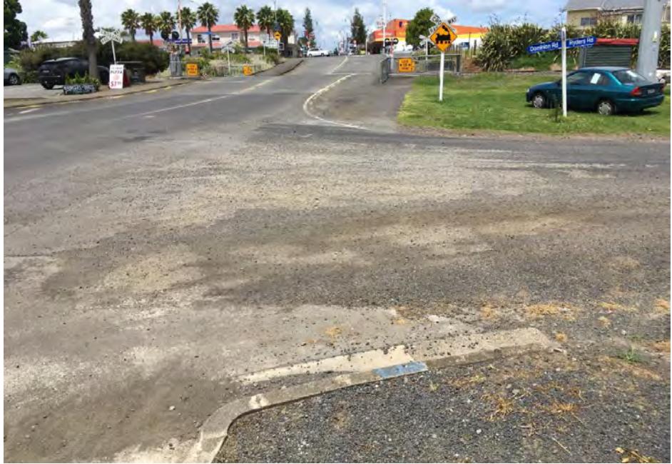
Looking towards the CBD. Note loose chip and little guidance.
