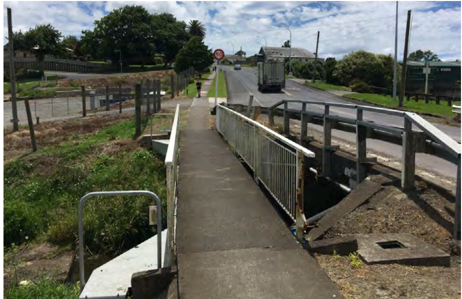
Separate walkway bridge on downstream side
