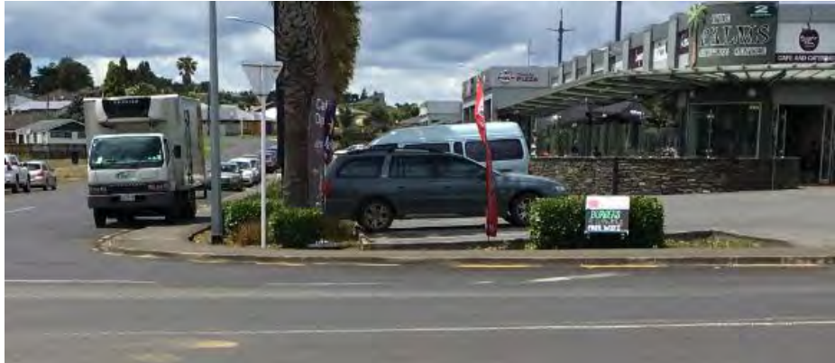
Looking east across George St. Lacks guidance as no pram crossing Where there is kerb and channel and a concrete footpath behind (south-eastern corner) there is no pram crossing kerb drop down to cross in either direction.
