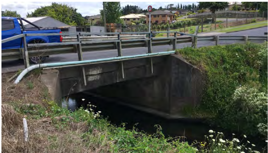
Potential footpath stream crossing from upstream on left streambank.
