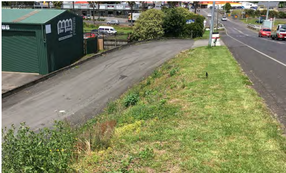
Steep bank into Miller Motors property
