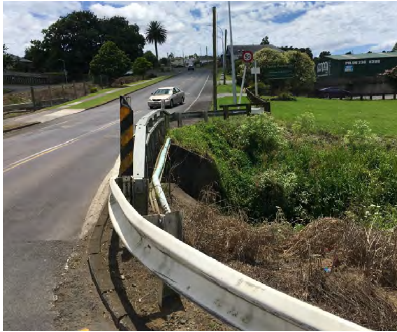
Looking uphill from south of Harrisville Rd Bridge
