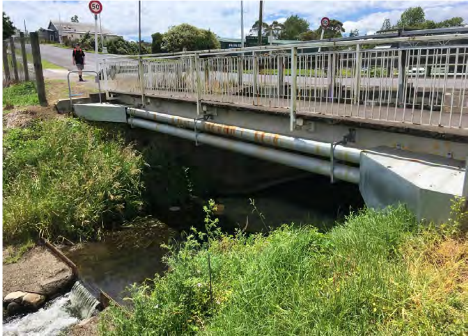
Downstream footbridge used for watermains also
