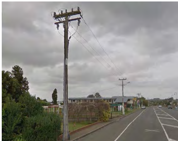
Poles on GSR to be removed and overhead lines undergrounded to McDonald Rd.
