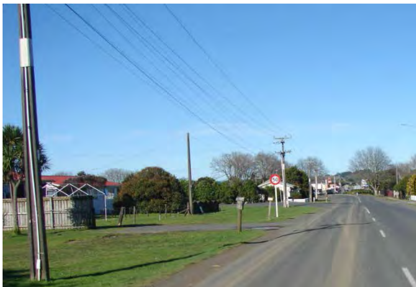
Poles on Pokeno Road to be removed and overhead lines undergrounded.
