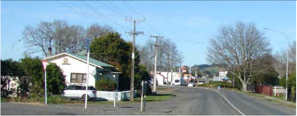
Poles on Pokeno Road and GSR to be removed and overhead lines undergrounded to Market St.
