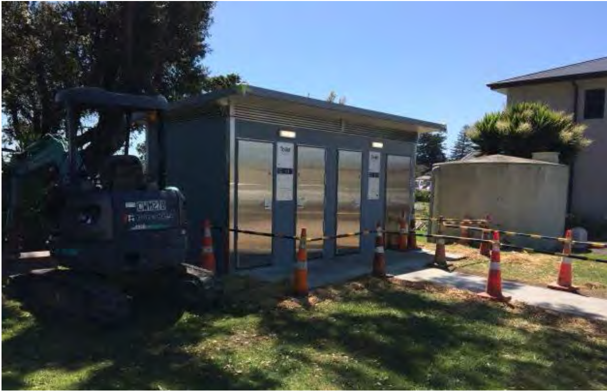
New Joyce Petchell Park toilet installed
