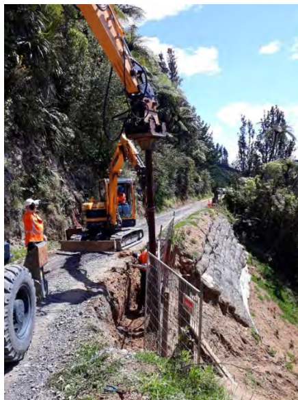
Installation of Railway Iron Retaining Wall on Klondyke Road
