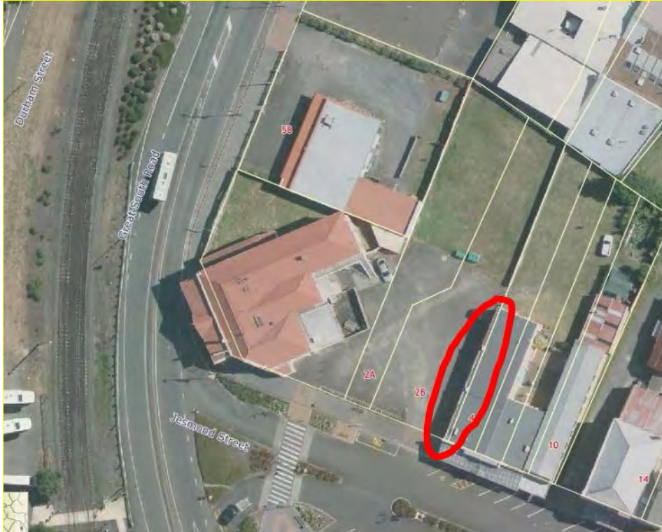
Ngaruawahia Library – western wall encroaches neighbouring property
