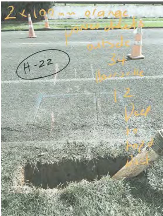
Tuakau Bulk main - Potholing
