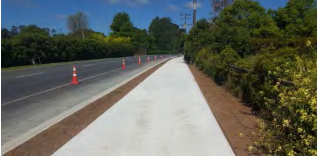
Tamahere Walkway/Cycleway – part of the Te Awa Cycleway
