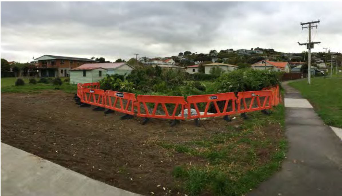
Stormwater Works completed at corner Wainui Road and Stewart Street
