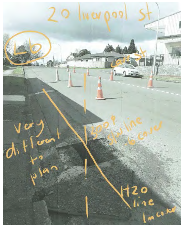
Potholing reveals services data to update design
