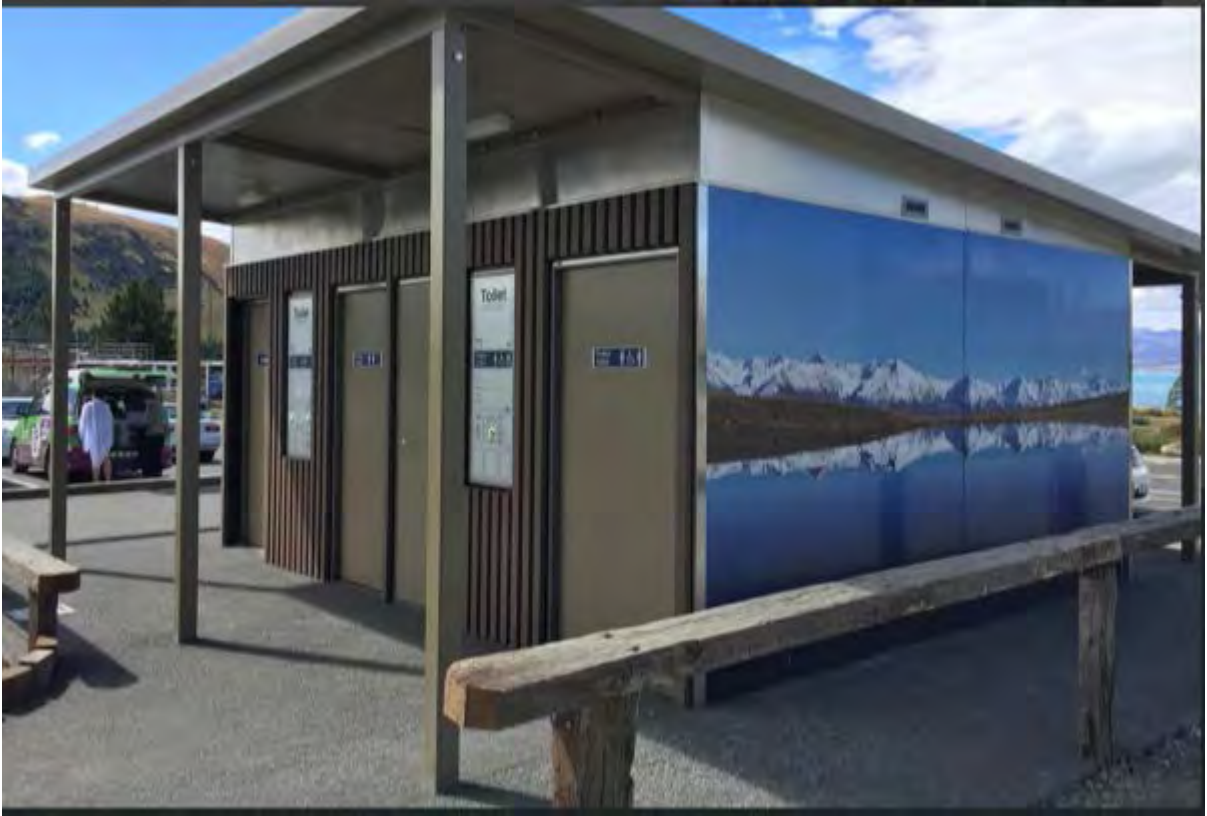
6 pan, extended roof on poles (both ends), wood batten and wrap finish – indicative costing for a 3 pan $166,500 - $176,500
