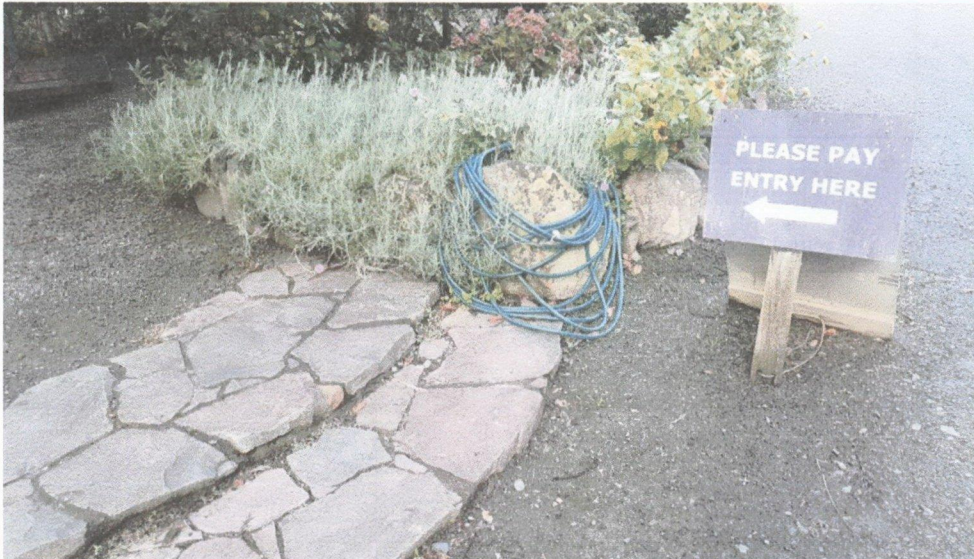
Photo 2: front steps leading to office may cause trips and/or falls (F27 on map)
