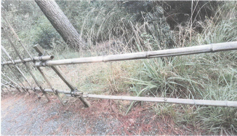
Photo 7: Bamboo fence at Folly is incomplete and batten showing is not stable
