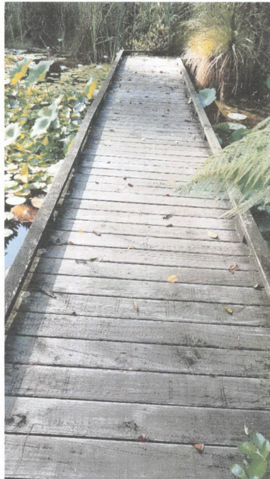
Photo 7: boardwalk, used for access and seating during events in quarry pond area
