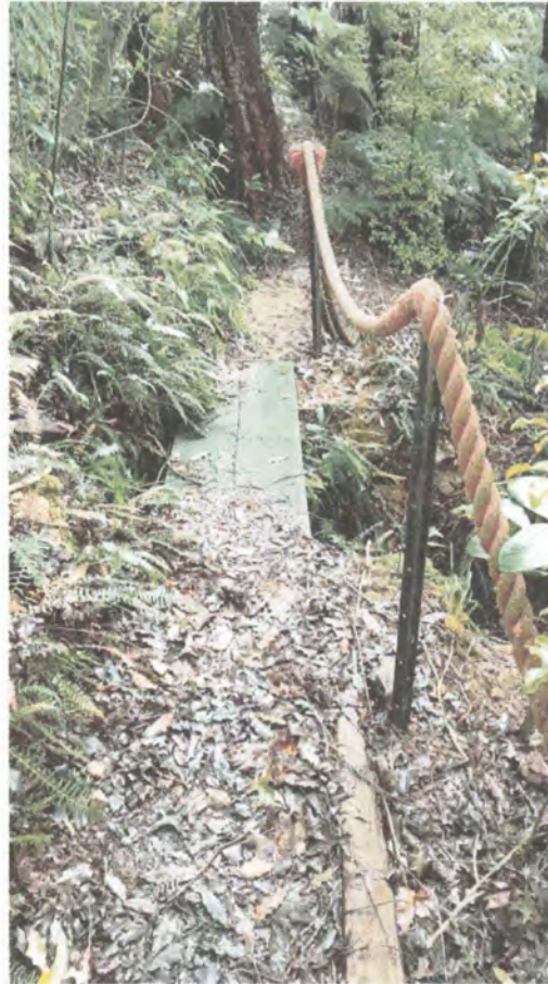
Photo 5: boardwalk over stream, rope hand guide
