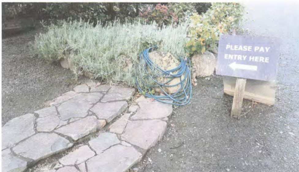
Photo 2: front steps leading to office may cause trips and/or falls (F27 on map)
