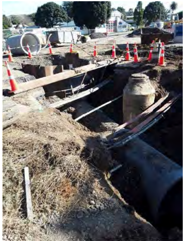
Significantly challenging Drainage works with multiple services and depths involved
