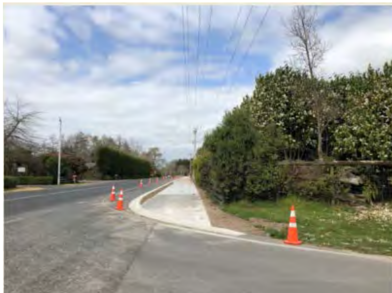
Newell Road Shared Path Progress Photo
