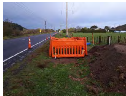
Pressure Testing underway for Hopuhopu to Huntly
