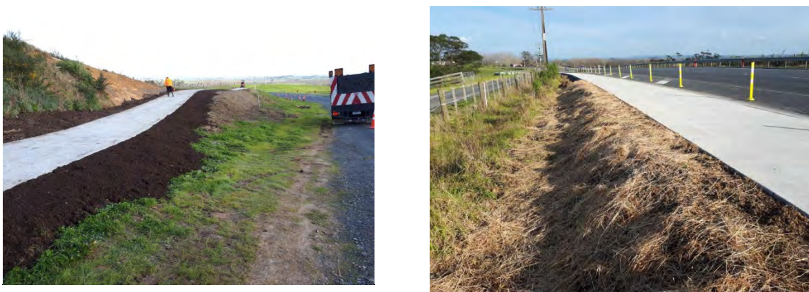
Te Kauwhata to Rangiriri Shared Path (Te Wharepu Rd) – finishing touches 05/07/2018
