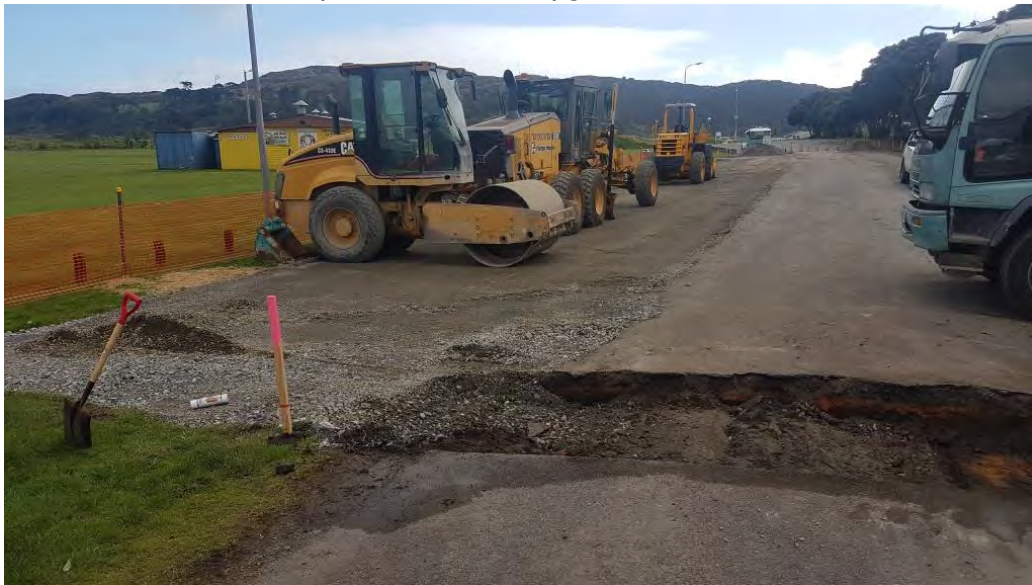
Papahua – Car Park Upgrade Works underway 10/08/2018
