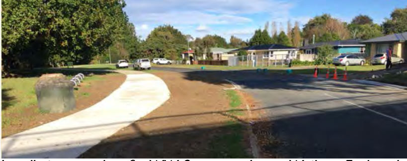
Installation complete for WW Storage at Lower Waikato Esplanade
