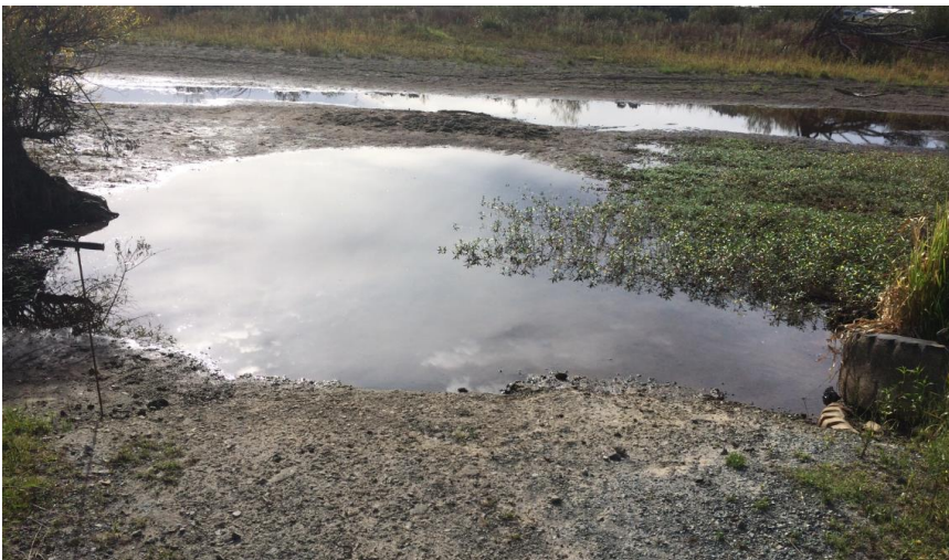
Figures 13 and 14: Channel siltation at the Riverview Road Boat Ramp, Waikato River restricting usage.
