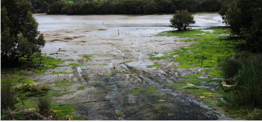
Figure 11: Gravel wash and siltation at Waingaro Landing Boat Ramp, Waingaro River
