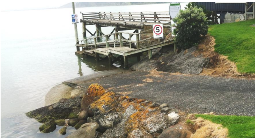
Figure 4: Port Waikato Boat Ramp with associated access platform/jetty.
