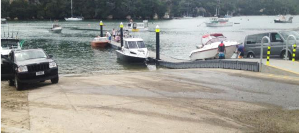
Figure 32: Upgraded Whitianga Boat Ramp Facilities
