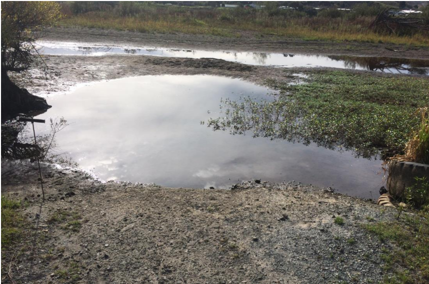
Figure 25: Launching point at the River Road boat ramp in Huntly West showing channel siltation and limited flows through this backwater channel compromising boat access.
