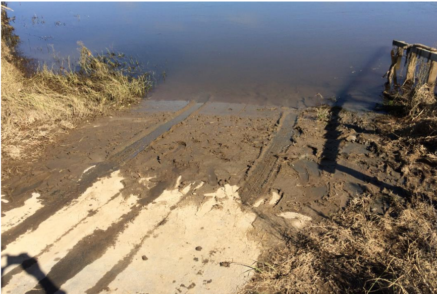
Figure 12: Heavy siltation following a recent flood event at Taupiri Boat Ramp, Waikato River
